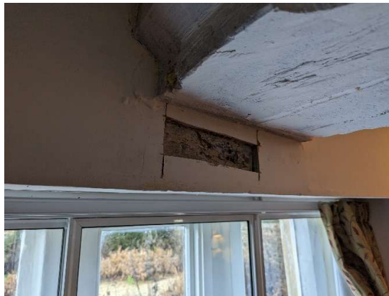
Figure 12: Photo of timber beam on concrete lintel
