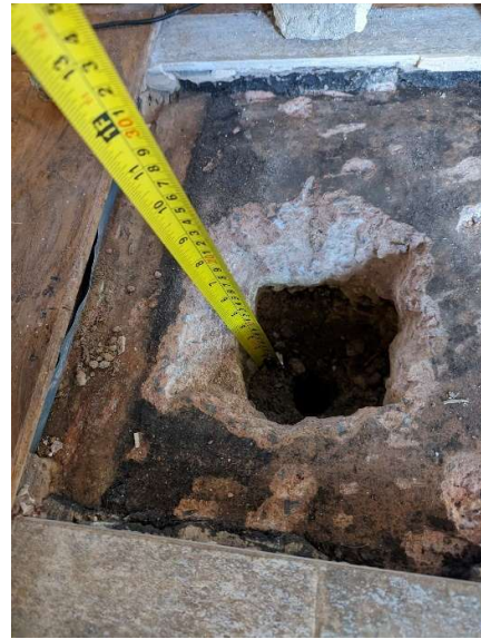
Figure 16: Photo of ground bearing slab
