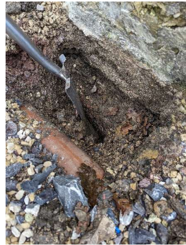
Figure 3: Photo of widened wall footing at trial pit location
