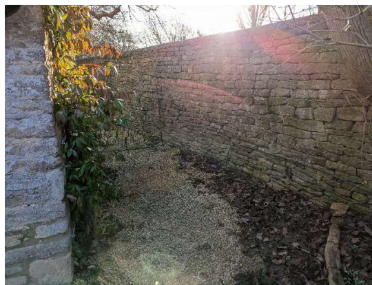
Figure 7: Photo of boundary wall
