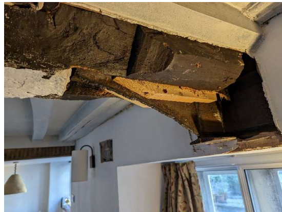
Figure 11: Photo of timber beam steel end connection
