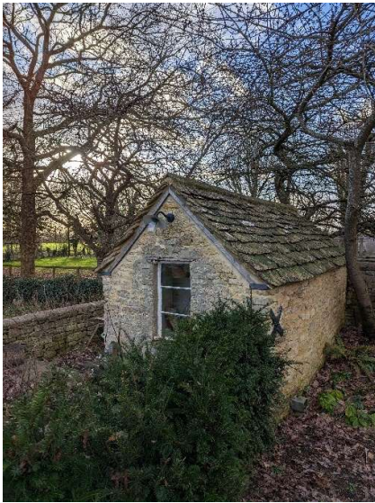
Figure 22: Photo of small outbuilding
