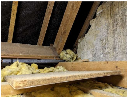
Figure 20: Photo of principle truss and purlin within loft
