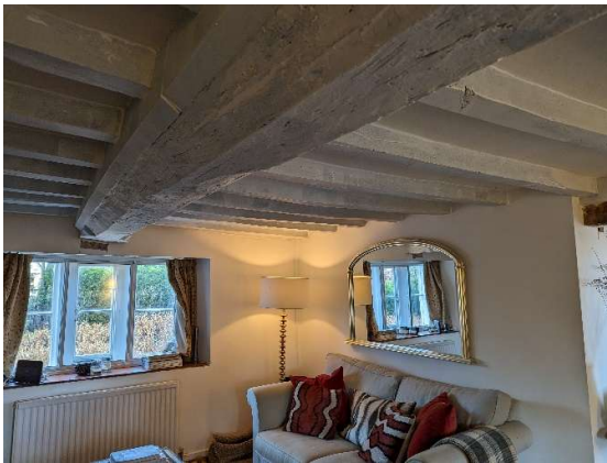
Figure 10: Photo of first floor joists and main timber beam
