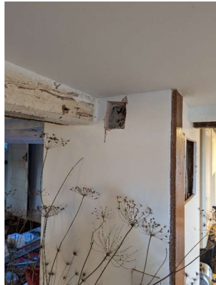
Figure 14: Photo of kitchen partition wall
