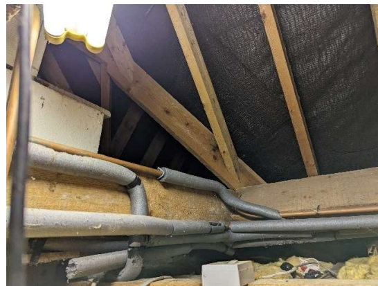
Figure 21: Photo of principle truss, purlin and valley beam within loft
