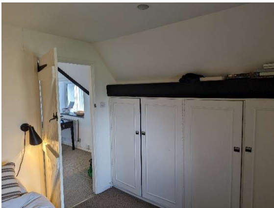
Figure 17: Photo of exposed purlin at first floor
