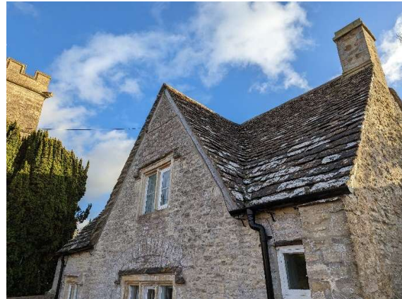
Figure 9: Photo of front gable and roof structure
