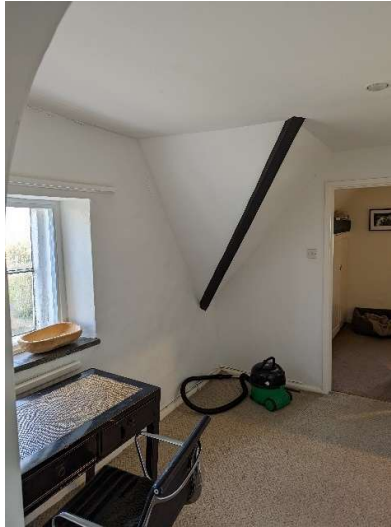
Figure 19: Photo of exposed valley beam
