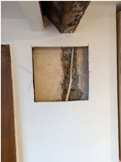
Figure 13: Photo of kitchen partition wall
