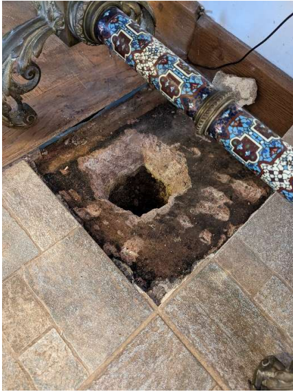
Figure 15: Photo of ground bearing slab
