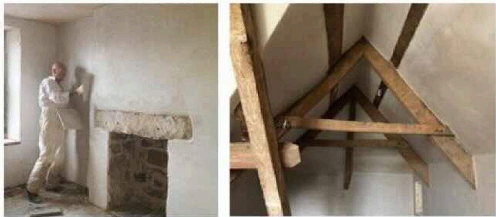
Hand trowelled Lime & Cork internal plaster finish
