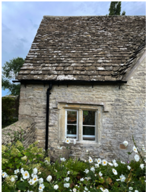
Existing roofing materials to be retained and reused in diminishing courses. Any additional roofing material to match existing natural stone. Valley details on outbuilding to be completed in stepped lead detail
