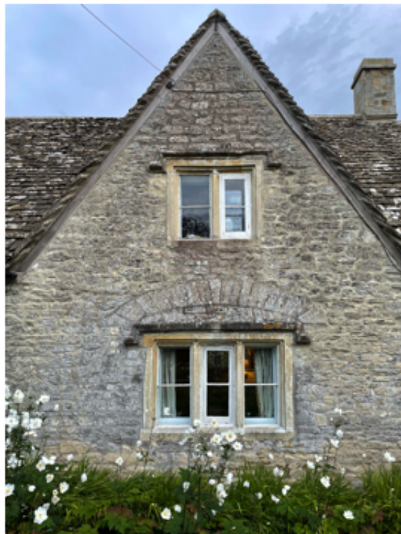
Any new natural stone to match existing appearance, from reclaimed local stone merchant Allow for lime pointing throughout Any work to external boundary wall to be completed in matching stone and laid in un pointed courses
