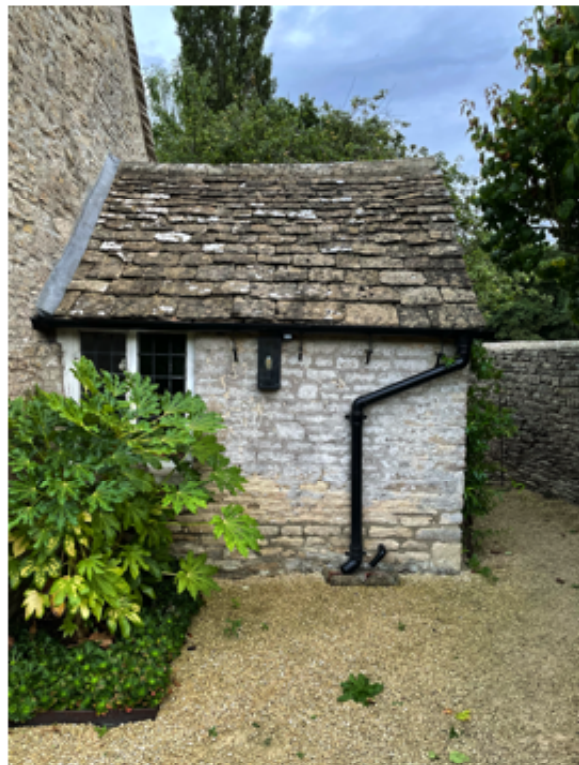
Existing roofing materials to be retained and reused in diminishing courses. Any additional roofing material to match existing natural stone. Valley details on outbuilding to be completed in stepped lead detail
