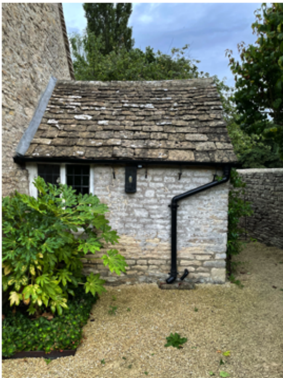
Any new natural stone to match existing appearance, from reclaimed local stone merchant Allow for lime pointing throughout Any work to external boundary wall to be completed in matching stone and laid in un pointed courses
