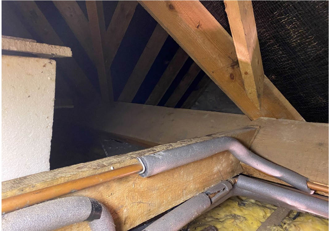
Figure 16: The roof structure viewed from the access hatch looking towards the southern gable structure.
