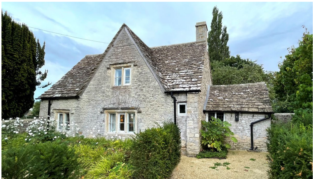
Figure 8: The Latchets front elevation, note projection of the western gable just right of the small stair window beneath the chimney.
