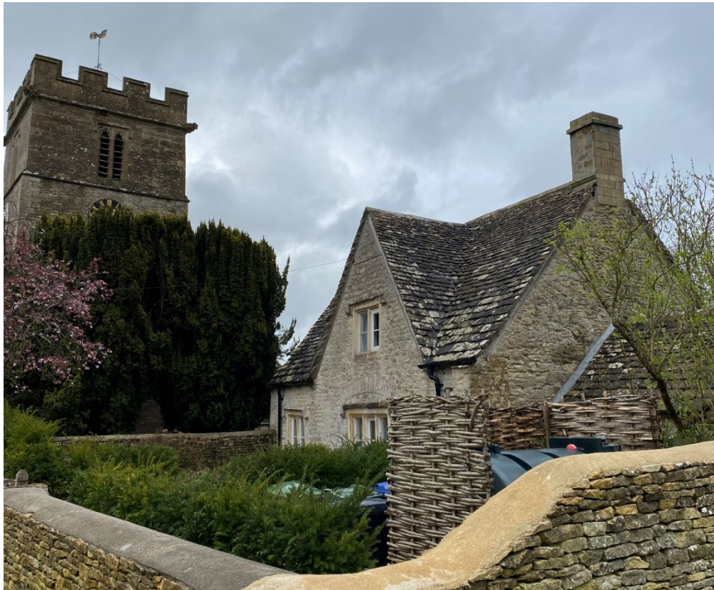
Figure 2: Latchets, north and western gable showing proximity to parish church.
