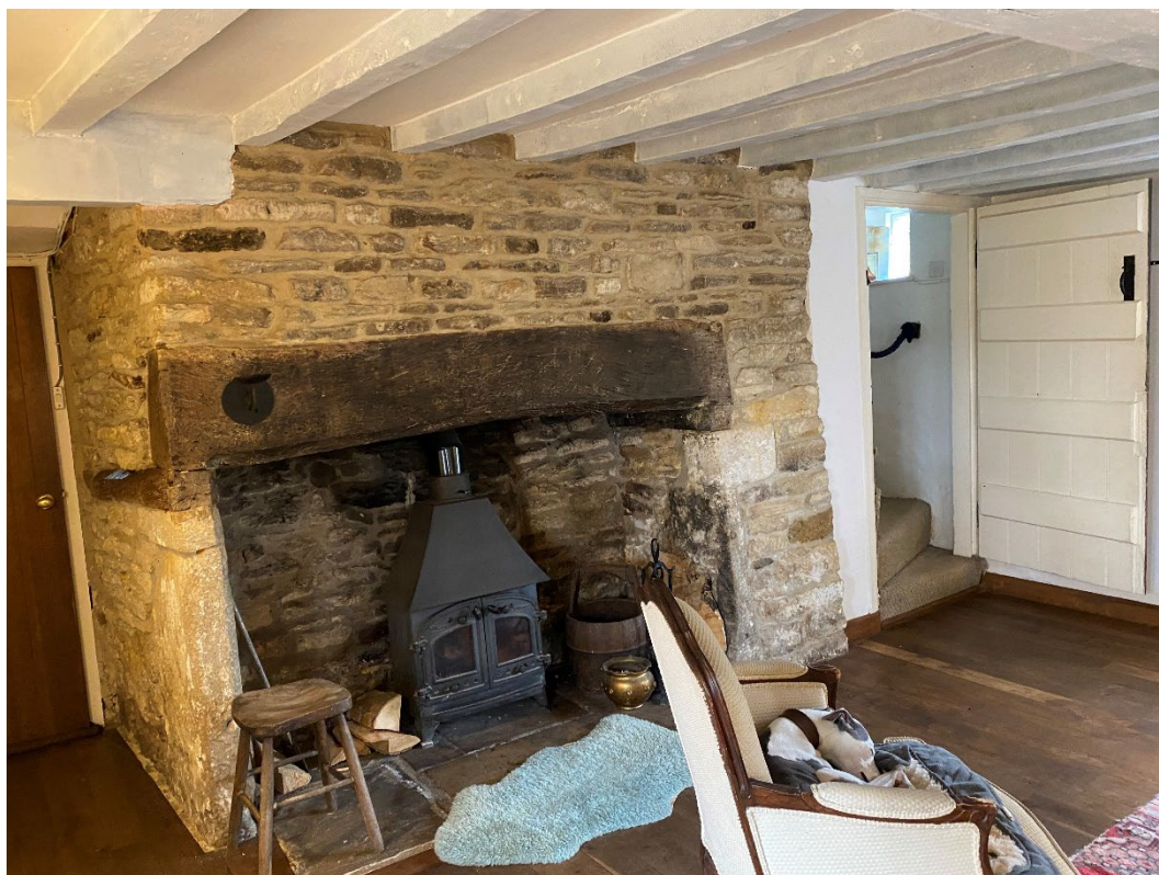
Figure 11: The large fireplace with timber bressumer and solid upright flanking stones, exposed timber floor/ceiling structure and traditional newel stair within the depth of the stack.
