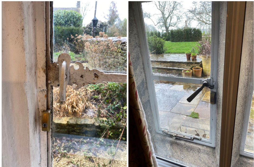
Figures 12-13: (left) surviving period iron casement with ornamental turn buckle catch lighting the kitchen and, (right) example of the type of 1930s style rolled steel casements seen elsewhere in the larger ground floor
