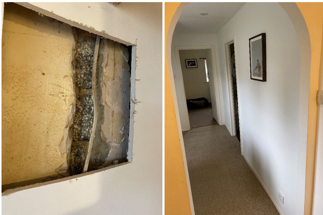
Figure 19-20: (left) typical material quality within downstairs area, this from within kitchen space and, (right) first floor corridor and all modern stud partition walls, to be altered with new layout.
