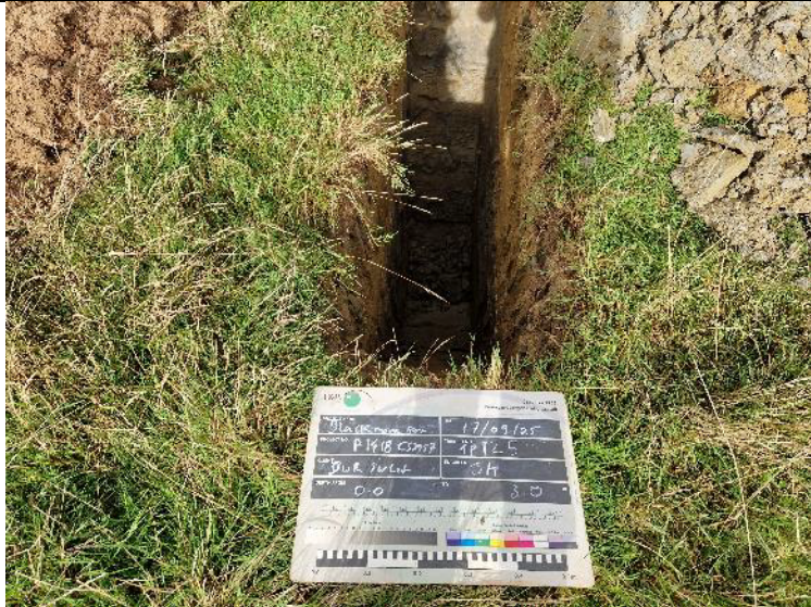
PLATE 49 – Trial Pit Excavation – TP125.
