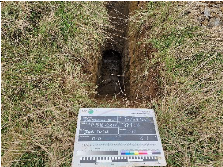
PLATE 55 – Trial Pit Excavation – TP128.
