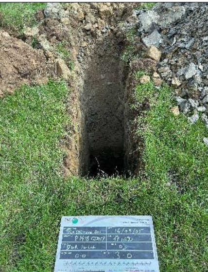
PLATE 43 – Trial Pit Excavation – TP122.
