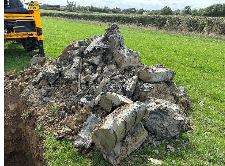
PLATE 46 – Trial Pit Spoil – TP123.
