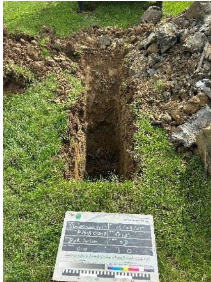
PLATE 45 – Trial Pit Excavation – TP123.
