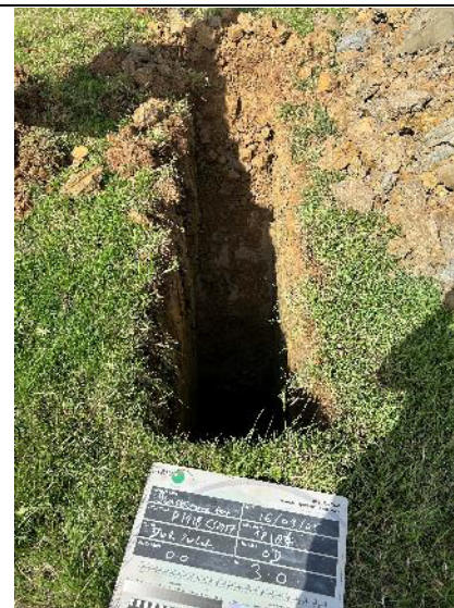
PLATE 47 – Trial Pit Excavation – TP124.
