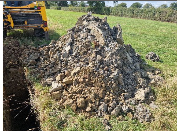
PLATE 38 – Trial Pit Spoil – TP119.
