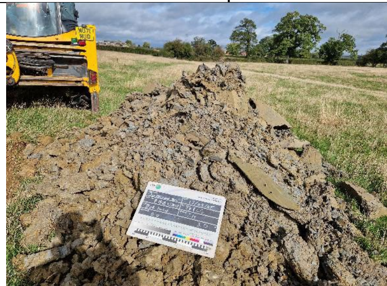
PLATE 52 – Trial Pit Spoil – TP126.
