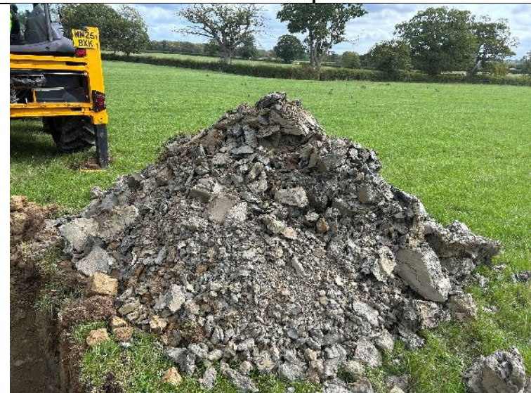
PLATE 44 – Trial Pit Spoil – TP122.
