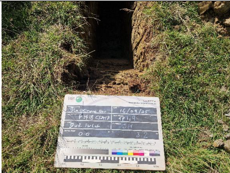
PLATE 37 – Trial Pit Excavation – TP119.
