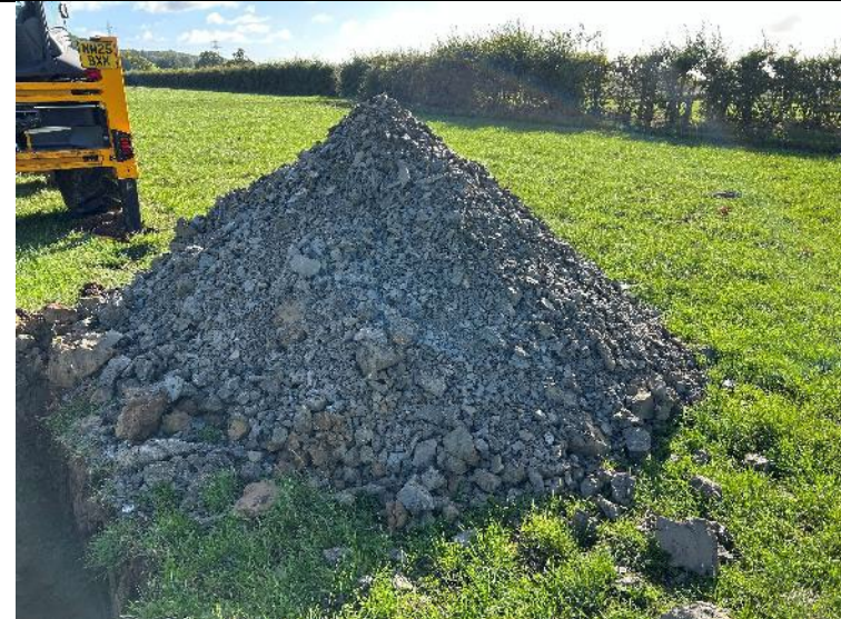
PLATE 06 – Trial Pit Spoil – TP103.
