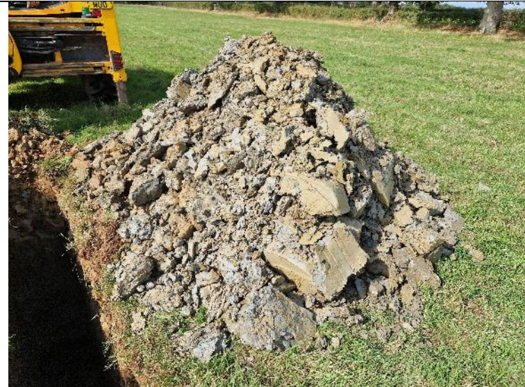
PLATE 30 – Trial Pit Spoil – TP115.
