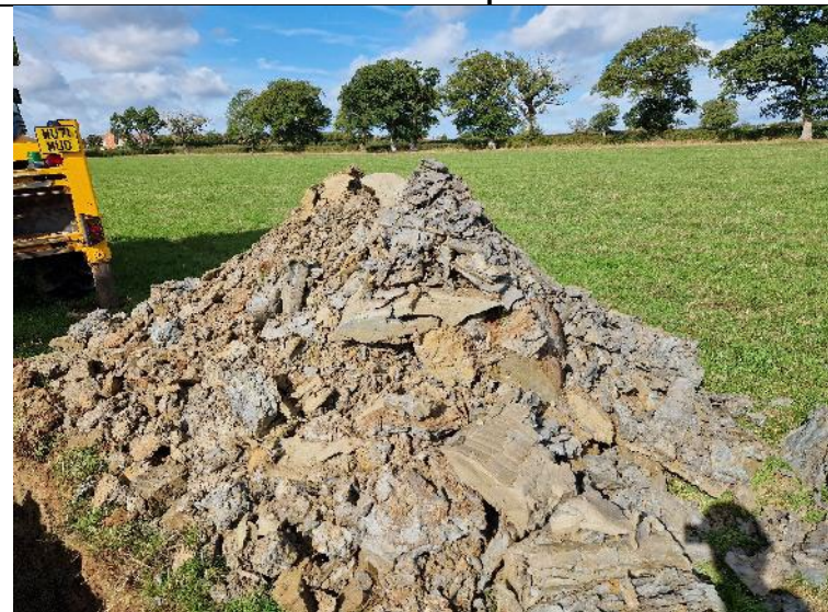
PLATE 28 – Trial Pit Spoil – TP114.
