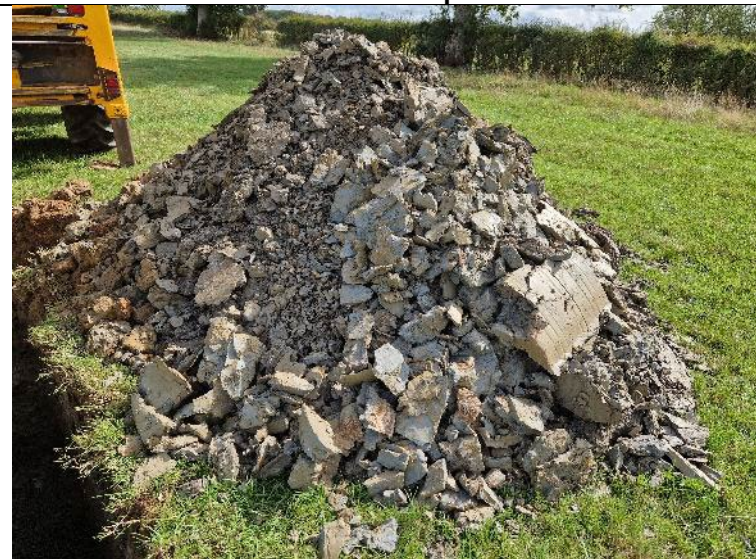
PLATE 32 – Trial Pit Spoil – TP116.
