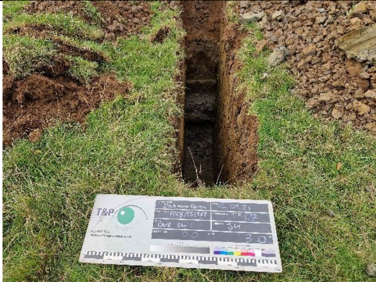
PLATE 33 – Trial Pit Excavation – TP117.
