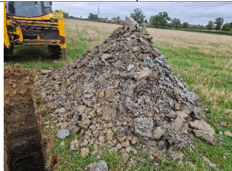
PLATE 16 – Trial Pit Spoil – TP108.
