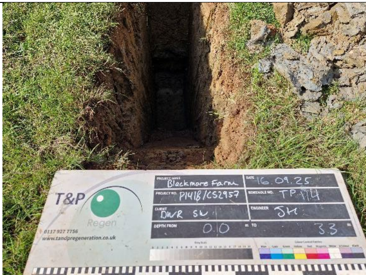
PLATE 27 – Trial Pit Excavation – TP114.
