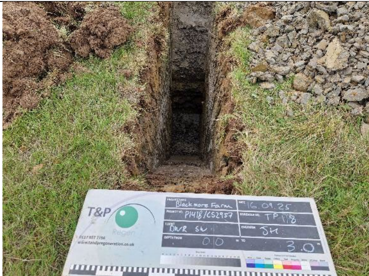
PLATE 35 – Trial Pit Excavation – TP118.
