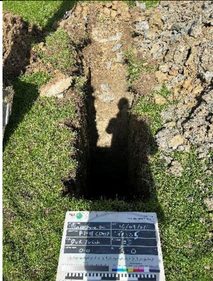
PLATE 09 – Trial Pit Excavation – TP105.
