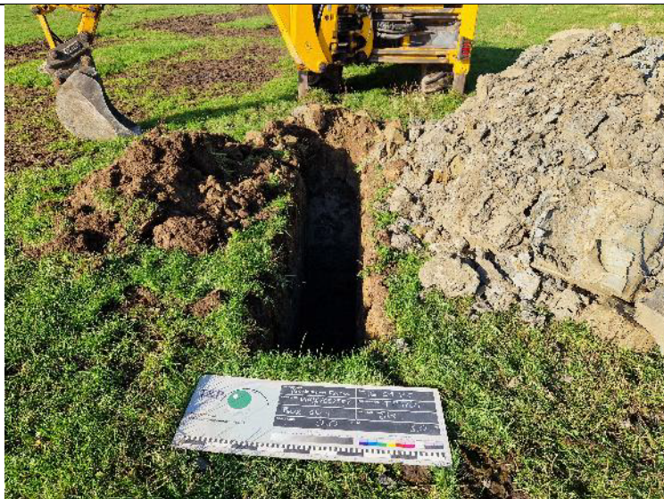
PLATE 03 – Trial Pit Excavation – TP102.
