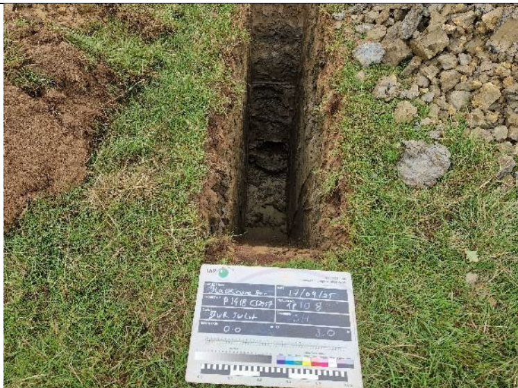
PLATE 15 – Trial Pit Excavation – TP108.
