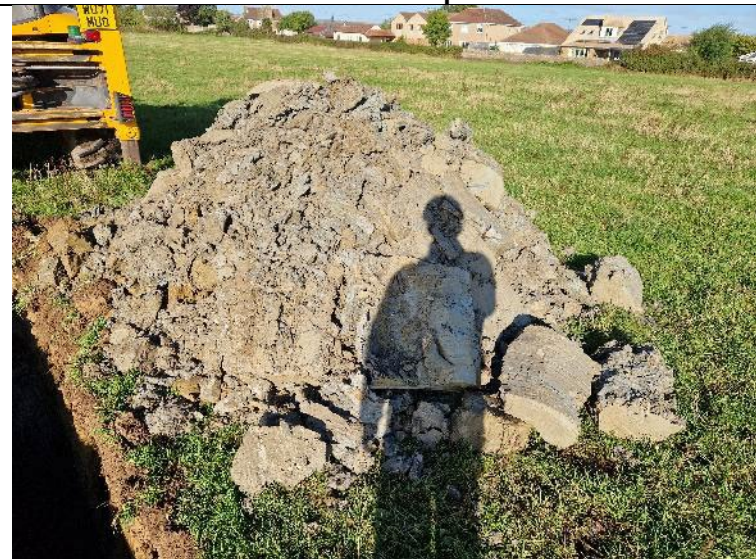
PLATE 04 – Trial Pit Spoil – TP102.
