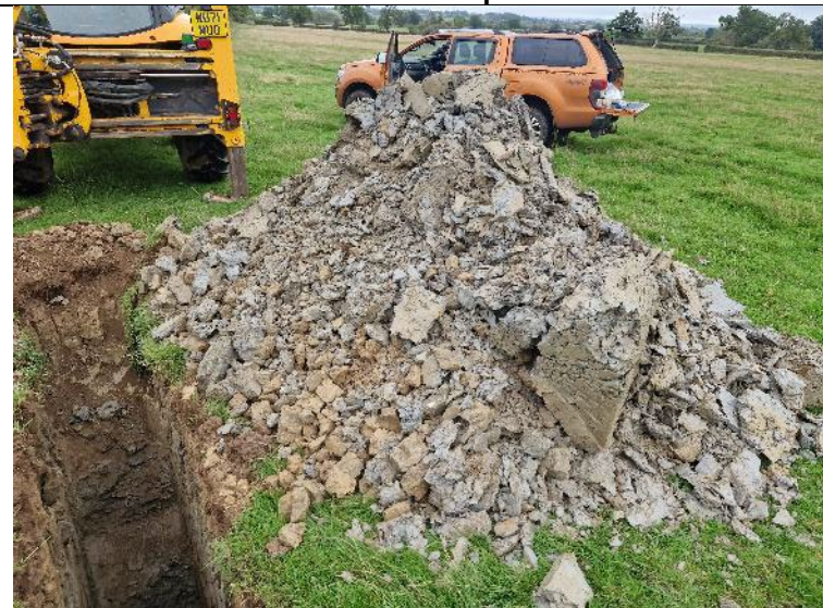
PLATE 08 – Trial Pit Spoil – TP104.
