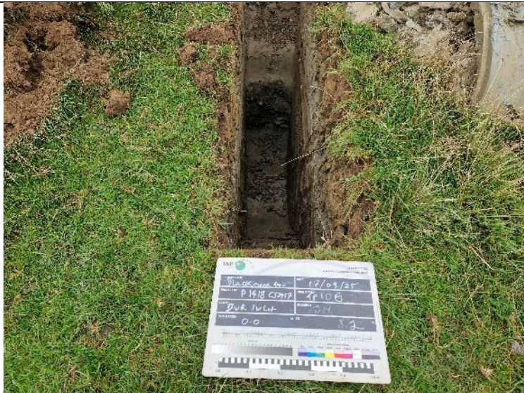
PLATE 11 – Trial Pit Excavation – TP106.
