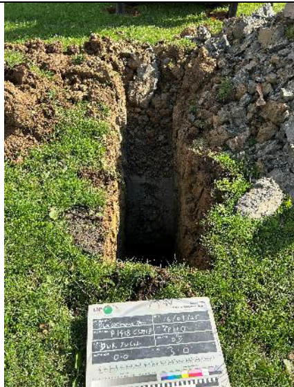
PLATE 19 – Trial Pit Excavation – TP110.
