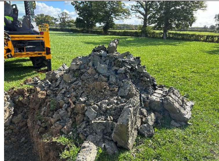
PLATE 20 – Trial Pit Spoil – TP110.
