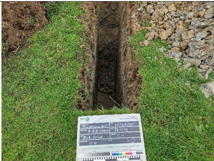
PLATE 07 – Trial Pit Excavation – TP104.
