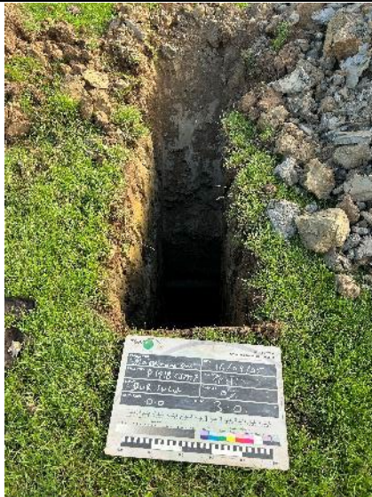
PLATE 21 – Trial Pit Excavation – TP111.
