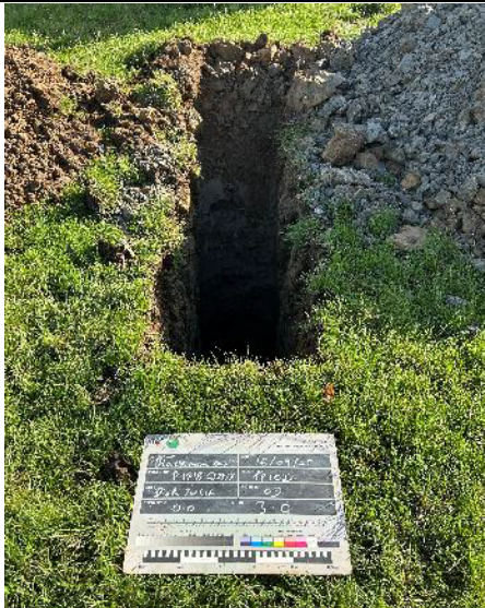
PLATE 05 – Trial Pit Excavation – TP103.
