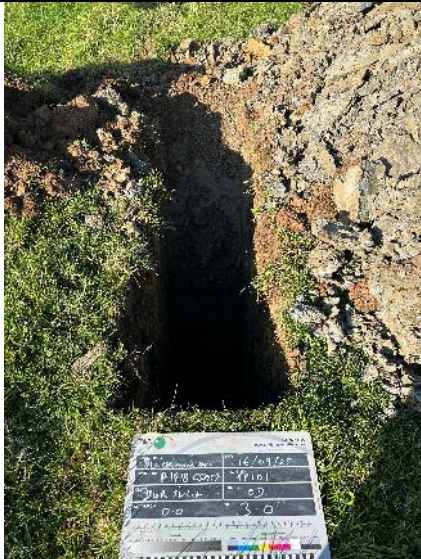
PLATE 01 – Trial Pit Excavation – TP101.
