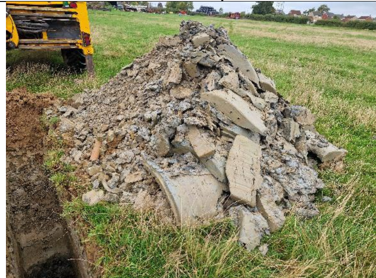
PLATE 12 – Trial Pit Spoil – TP106.
