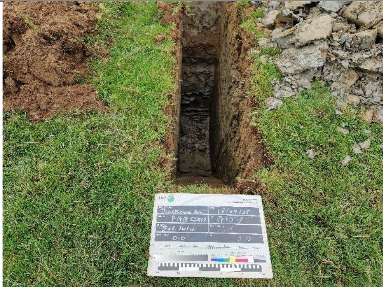
PLATE 13 – Trial Pit Excavation – TP107.
