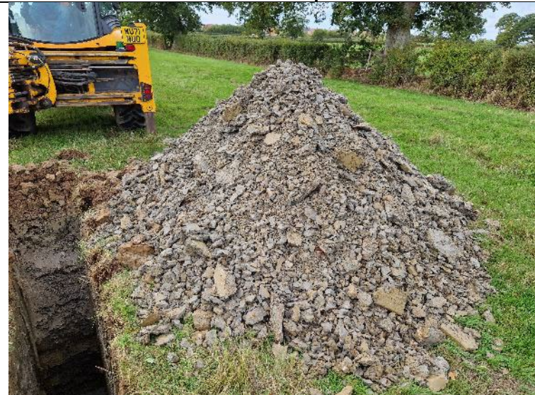
PLATE 36 – Trial Pit Spoil – TP118.
