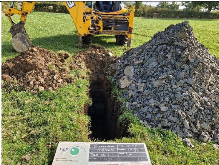
PLATE 23 – Trial Pit Excavation – TP112.
