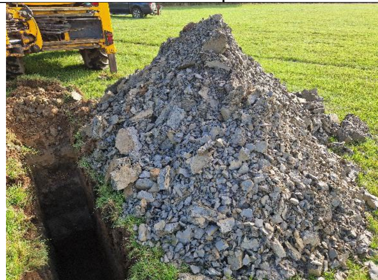
PLATE 24 – Trial Pit Spoil – TP112.
