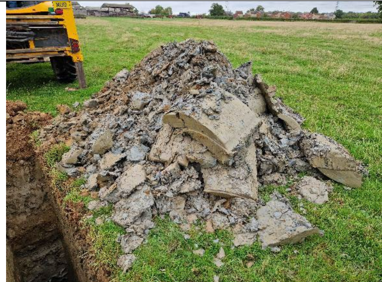
PLATE 14 – Trial Pit Spoil – TP107.
