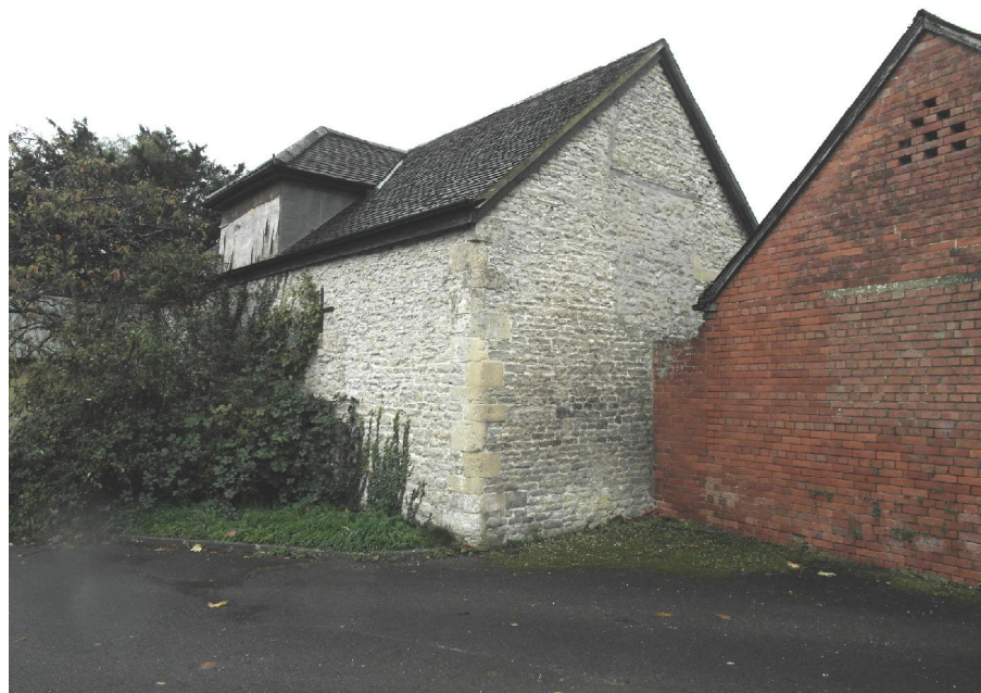
4. The eastern gable elevation of the barn which lies on the northern side of the main entrance into the Fives Court complex. Possible blocking shown by wooden lintel may indicate a former doorway giving access to an upper floor. The barn dates to before 1821. View to north-west.
