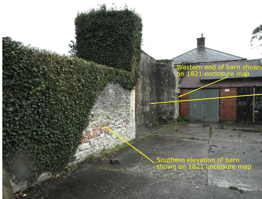
5. The so-called Fives Court Wall, which is a Grade II Listed structure. The element on the left may well be the southern elevation of a barn that was present in 1821. View to north-east.
