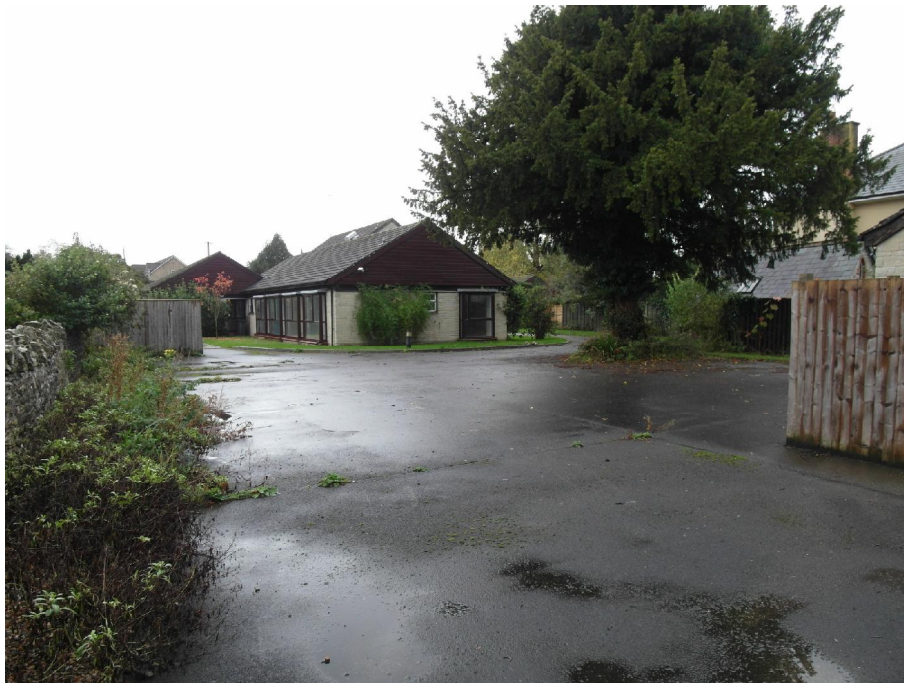
2. View of the site from the northern car park, close to its north-eastern corner, looking south-west.
