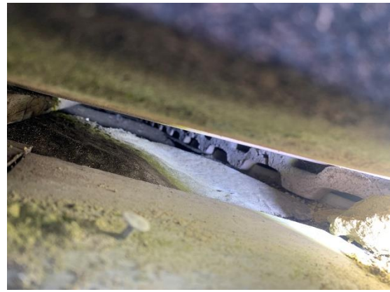
Photo 18 Internal cavity of PRF2. Feature extends along the length of the lower eave
