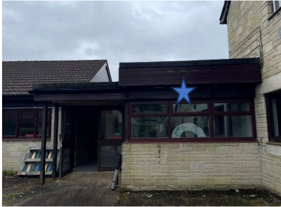
Photo 15 Western elevation of building with entry/ exit feature in the soffit (PRF – flat roof void over ground floor room)
