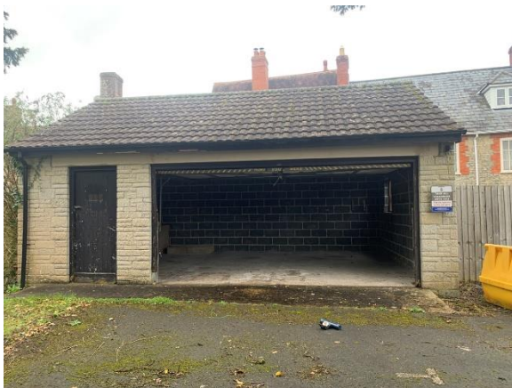
Photo 21 Southern elevation of the garage
