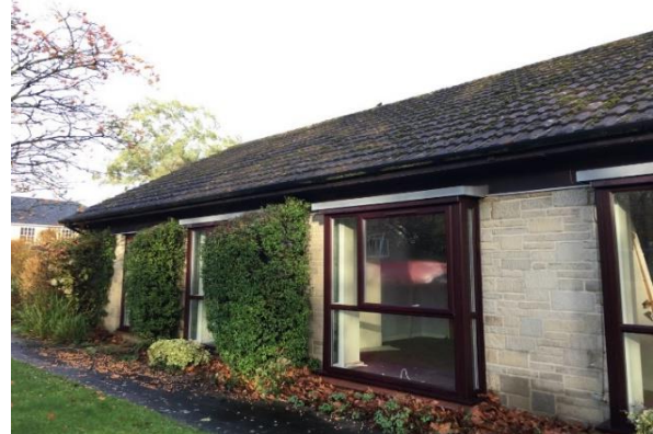
Photo 14 Eastern elevation of northern wing B1
