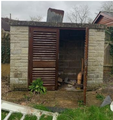
Photo 23 External of the gas building
