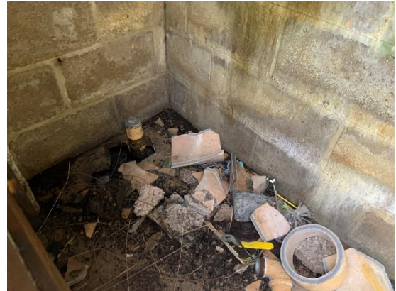
Photo 24 Internal of the gas building
