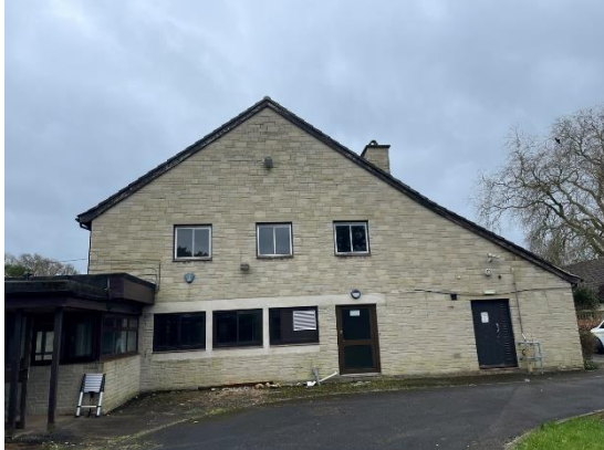
Photo 13 Northern elevation of two storey section of B1
