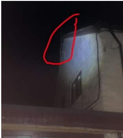
Photo 28, emergence location on southern elevation of two storey section - July.
