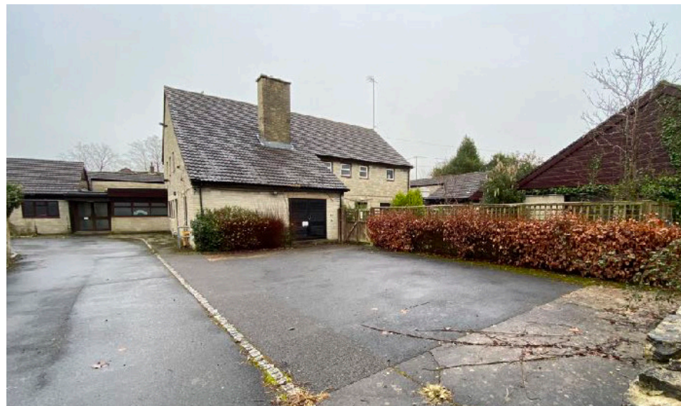
Existing access and dominance of plant room on approach
