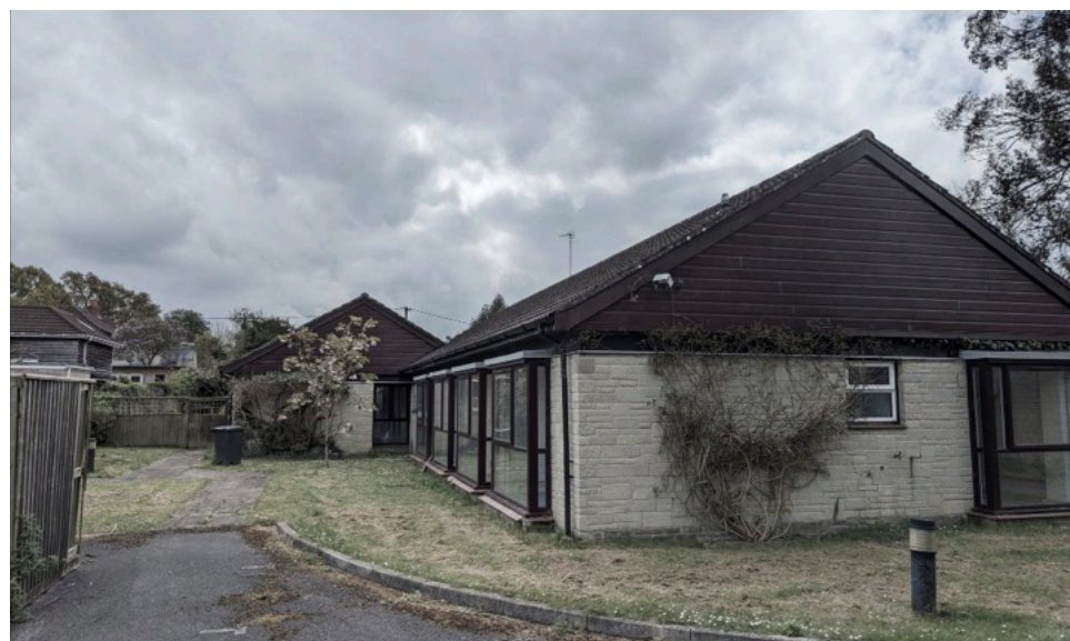
Existing building with the dressed North Cerney random course blockwork ground floor walls and timber clad gables above
