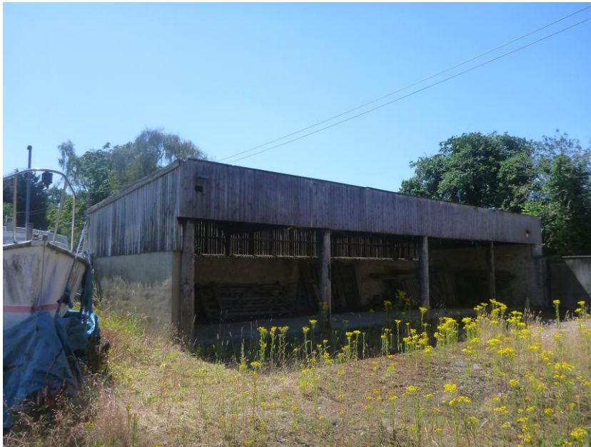
Fig 5: The open barn structure on the southern edge of the site.
