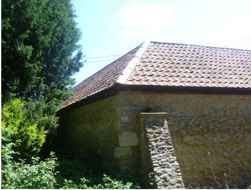
Fig 4: The north face of the stables.
