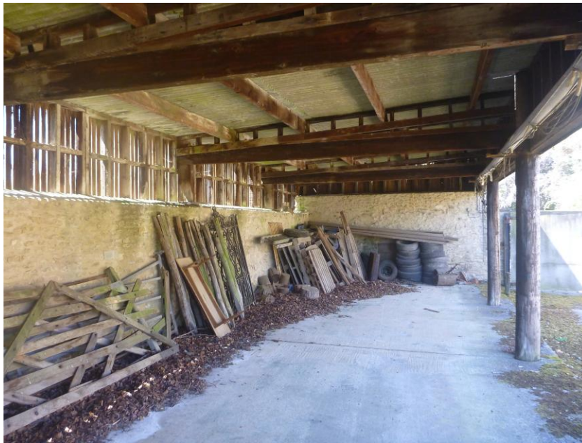
Fig 6: The open barn structure on the southern edge of the site.
