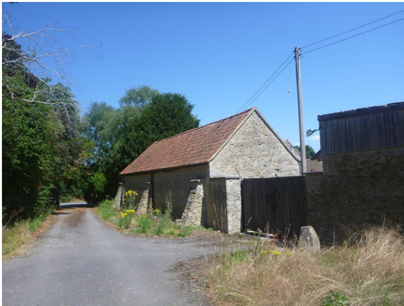
Fig 3: There are no doors or windows on the west or north aspects of the stable building.
