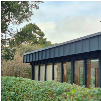
Coated Aluminium standing seam RAL 7015 Slate Grey - to facias of single storey flat roofs
