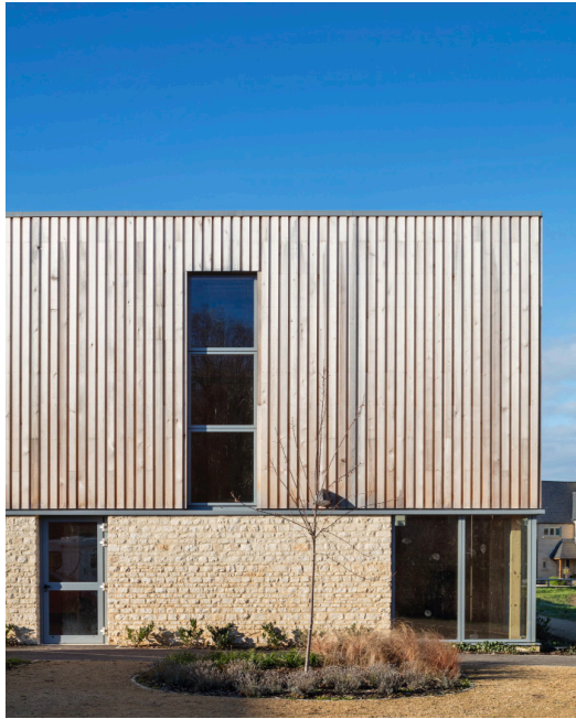
Cotswold stone ground floor and timber first floor - South Cemey
