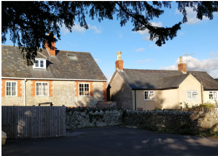
Rear of buildings north of the site
