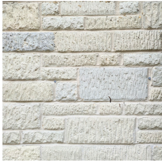
Existing Stonework Reconstituted / light sandstone mortar - retained stonework on the ground floor
