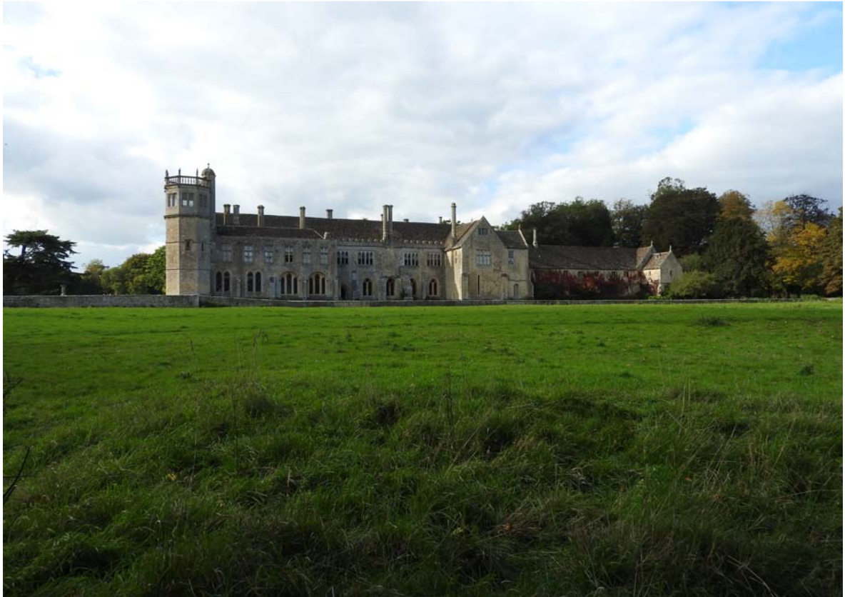
The East facing side of Lacock Abbey looking across 'Home Field'
