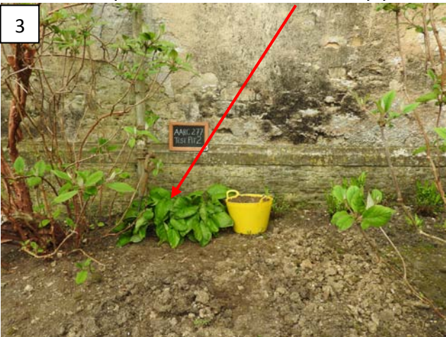
Test pit 2 next to the metal downpipe and drain and adjacent to the North facing wall
