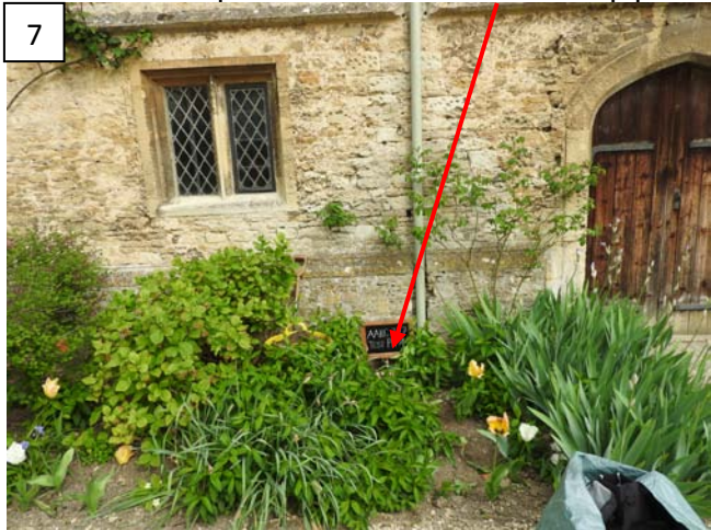
Test pit 4 next to the metal downpipe and drain and adjacent to the West facing wall
