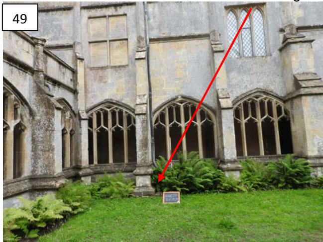
Test Pit 24 located to the right of the buttresing and drain
