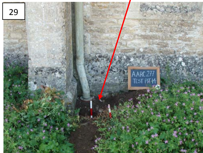
Test Pit 14 showing the downpipe and glazed collared pipe [1401]. Measures 2x0.3m
