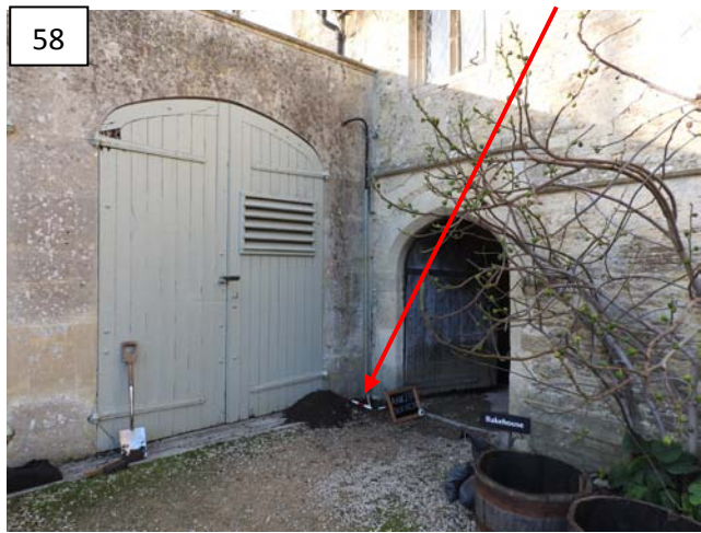
Test Pit 30 and electrical conduit and cable [3001]
