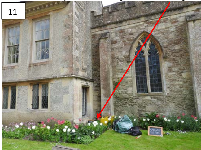
Test pit 6 cut through 0.3m of shingle/aggregate next to the outer kitchen
