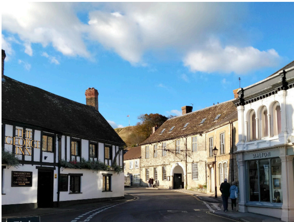
Listed buildings in Mere centre with the Scheduled Monument of Castle Hill in the background.
