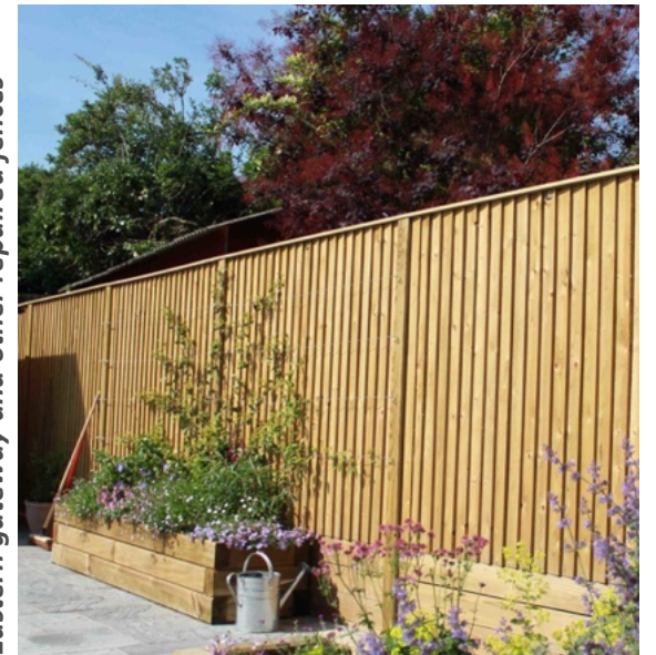
Proposed timber closeboard fencing - 1.8m high, pressure treated softwood, with matching gates.
