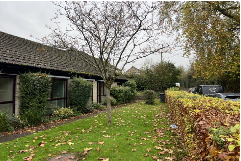
Photo 3- The lawn to the west of the building is contained by frontage hedgerows facing onto Angel Lane.
