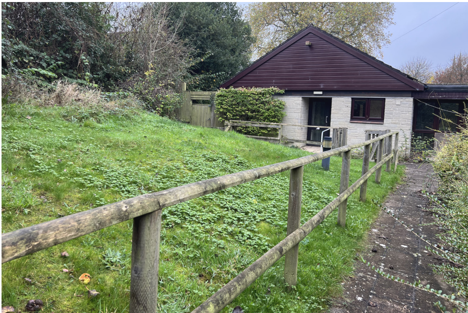
Photo 1- The grass area south of the building faces a steep upward slope and is enclosed by a post-and-rail fence.
