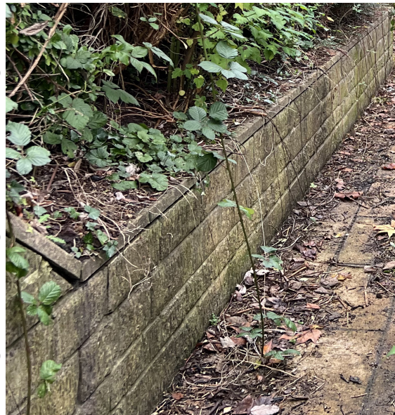
Existing concrete retaining wall to be retained, to be cleaned, vegetation cut back and coping re-set as necessary.
