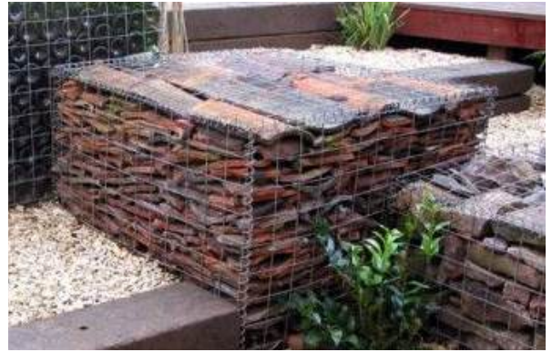
The picture above shows an example of reusing tiles to form retaining gabion walls.
