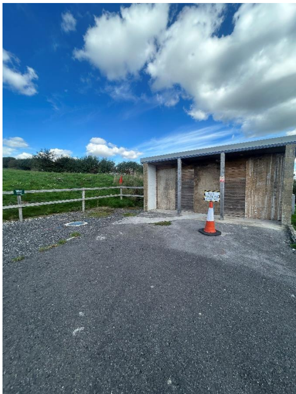
View of the toilet block looking north-east
