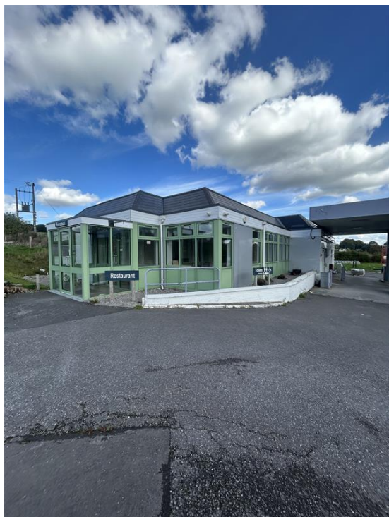
View of the existing petrol station looking north-east
