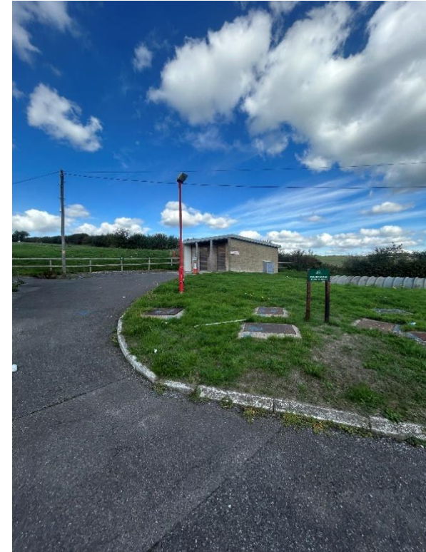
View of the toilet block and septic tank in eastern portion of the site.
