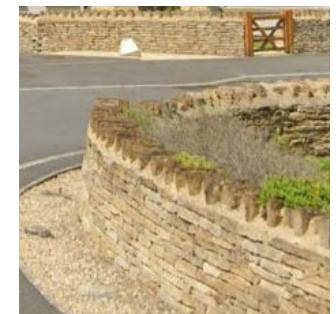
Dry stone boundary wall with vertical coping stone
