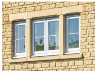
Stone lintel and sill
