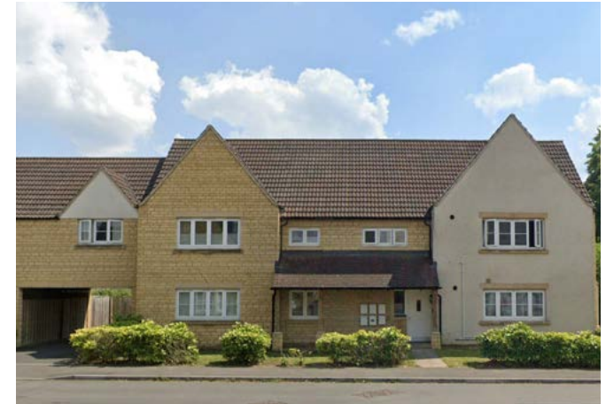
Continuous frontage, with breaks in the roofline and ground floor
