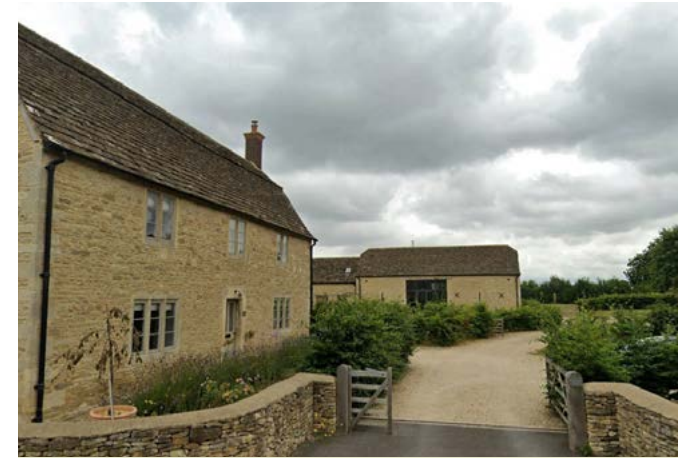
Arms Farm, converted stone farm building
