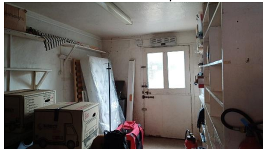
Photo 9 Ground floor internals
