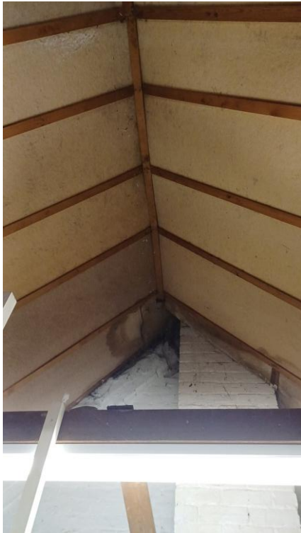
Photo 6 First floor ceiling
