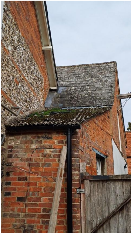
Photo 3 Rear of the structure
