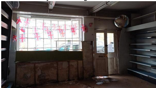
Photo 8 Ground floor internals
