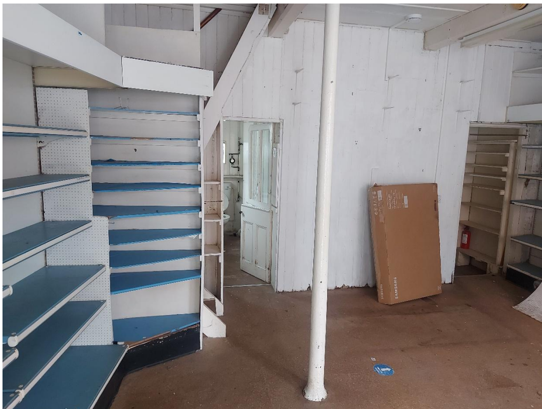
Figure 8: Internal view of rear of former shop
