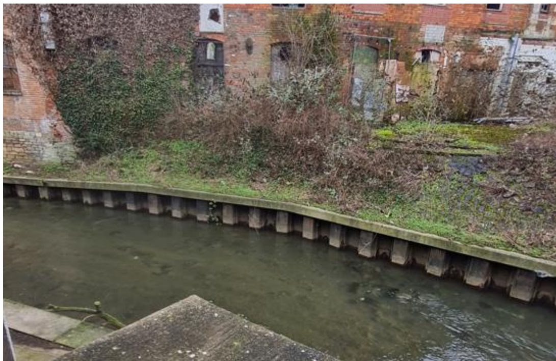
Figure 3-4 Flood Defences along River Biss
