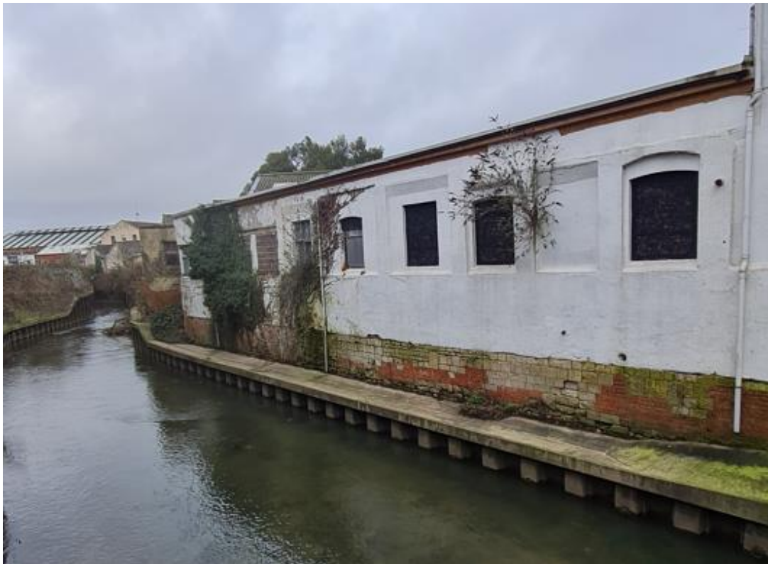
Figure 1-2 Existing Downpipes on building
