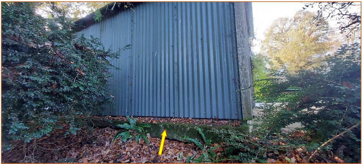
Image 5: The subbase of the existing pool house should be left in situ to avoid unnecessary root disturbance or carefully removed by hand to minimise harm
