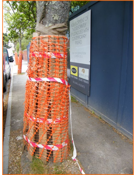
Pictures 4 & 5: Wooden boards carefully secured around the trunks can provide good protection where access is limited.
