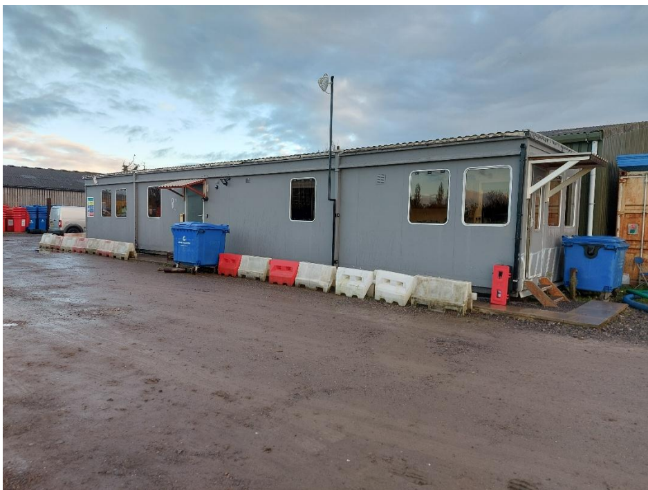
Figures 8 and 9: Views of office building in situ
