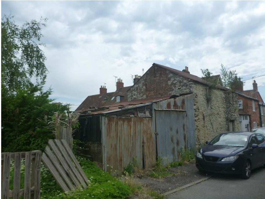
Fig 8: There is a single storey corrugated metal lean-to at the northern end of the barn.
