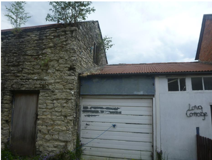
Fig 7: There is a single storey garage which links the barn to Long Cottage.
