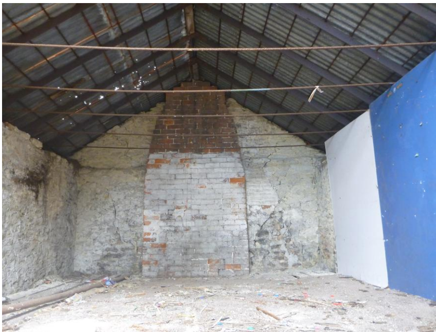
Fig 5: The roof is unlined corrugated metal.
