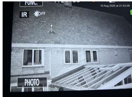
Photo 17: Example infrared camera view
