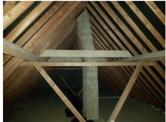
Photo 8: B1 - The single loft void covers the entire main section of the building.
