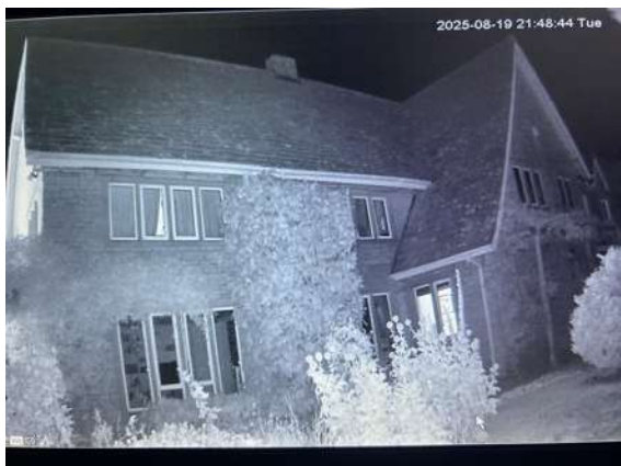
Photo 18: Example infrared camera view
