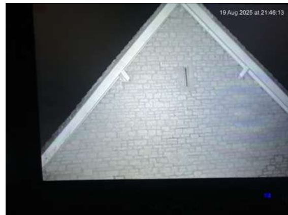
Photo 19: Example infrared camera view
