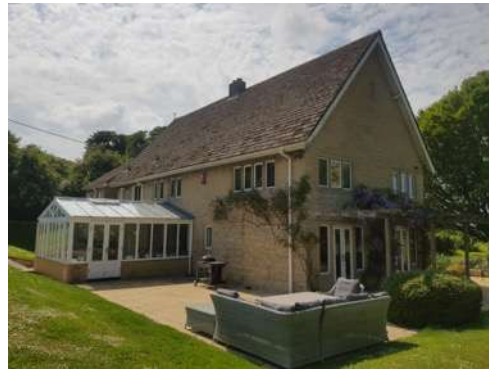
Photo 2: B1 - Dwelling viewed from the north
