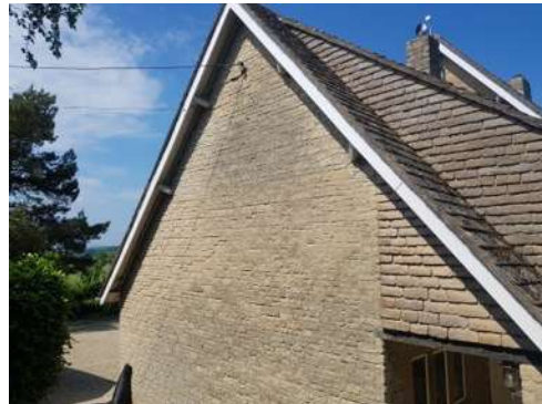
Photo 4: B1 - The south-east facing gable end wall.
