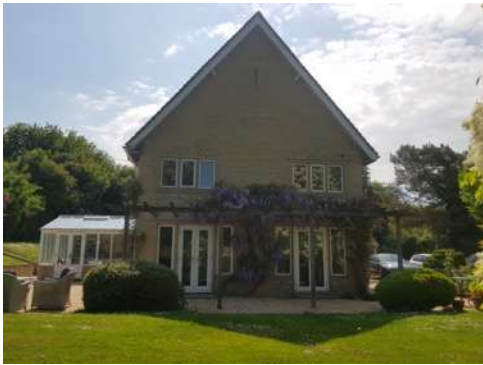
Photo 3: B1 - The north-west facing gable end of the dwelling
