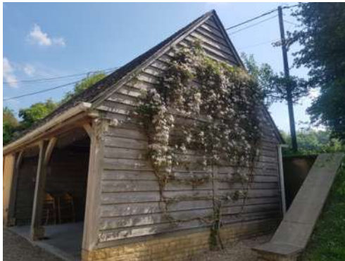
Photo 14: B2 - Timber cladding of garage structure
