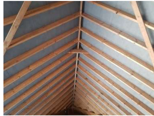
Photo 15: B2 - internal view of roof structure
