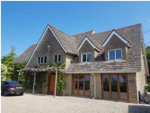
Photo 1: B1 - The roof of the dwelling is clad in imitation stone tiles
