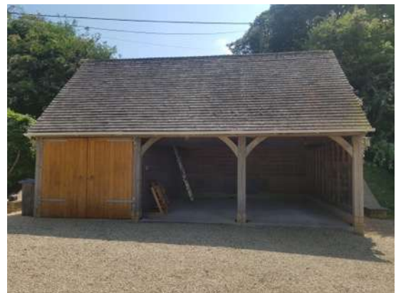
Photo 13: B2 - Garage structure
