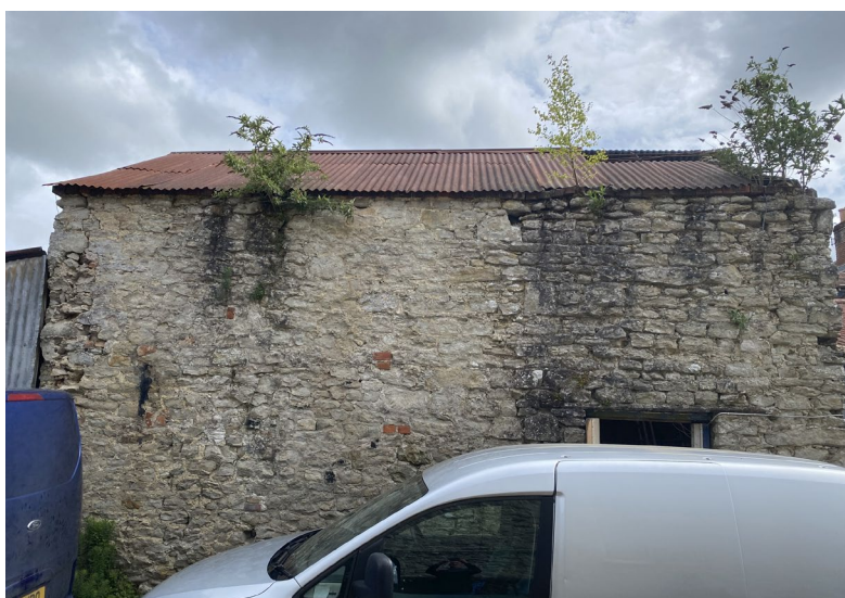
Stonework repairs and a new slate roof to the barn.
