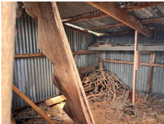
23: General interior of shed.
