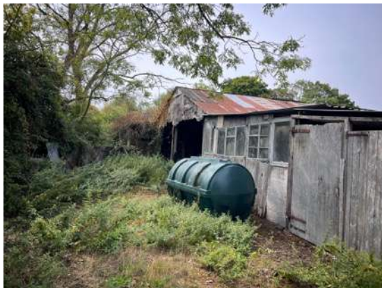
3: South elevation of the barn and view of hard standing colonised by nettle.
