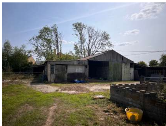
5: View of the north elevation of the barn.
