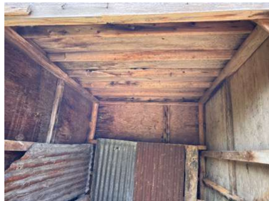
24: General interior of shed.
