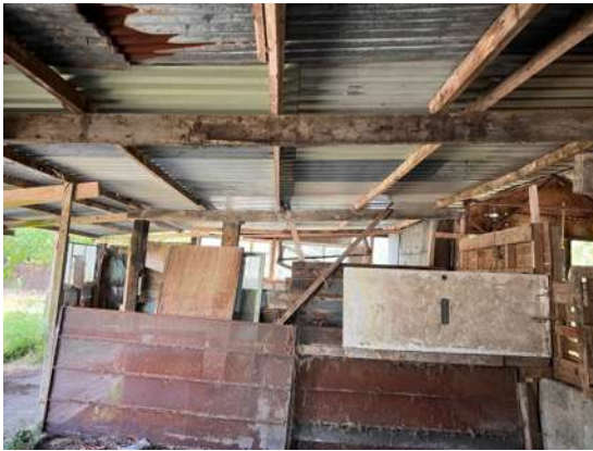
19: General interior of east section of the barn.
