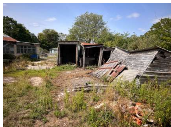
6: View of the sheds and surrounding hardstanding.
