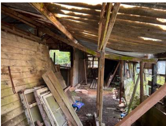
17: General interior of west section of the barn.
