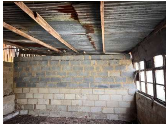
20: General interior of east section of the barn.
