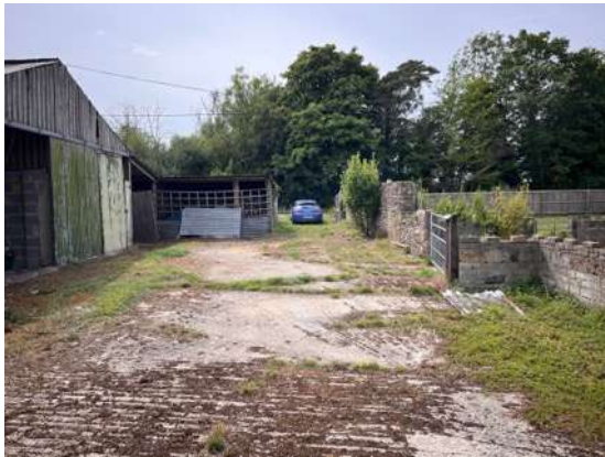
1: West facing view of the site.
