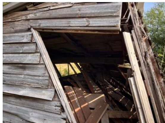
26: General interior of shed.
