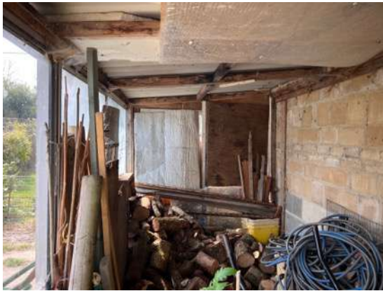
21: General interior view of the outbuilding.
