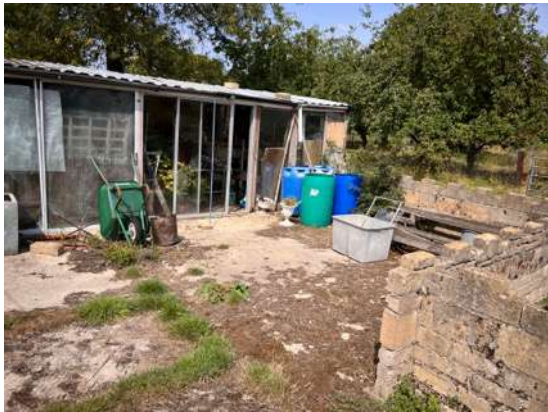
7: South elevation of the outbuilding.
