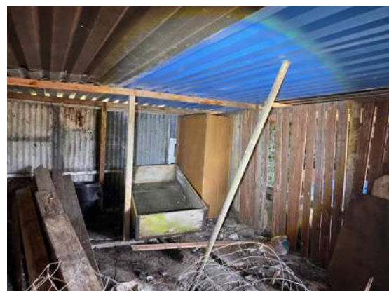
18: General interior of west section of the barn.
