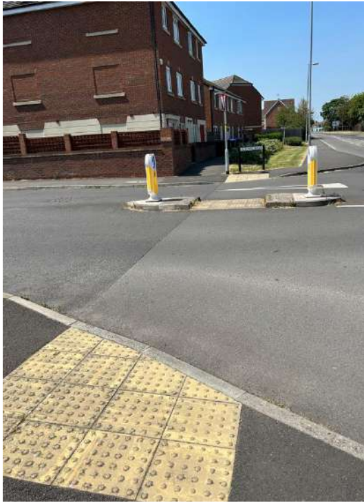
Photograph 6: Pedestrian infrastructure along Skylark Road junction
