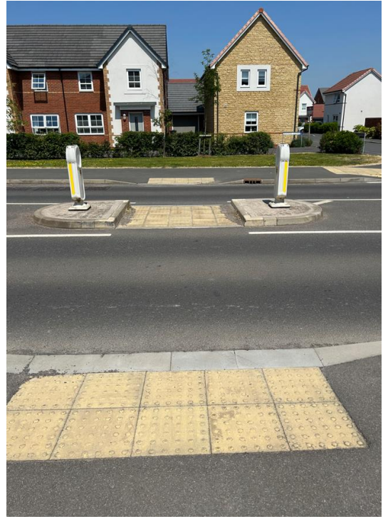
Photograph 7: Existing pedestrian crossing infrastructure along Sandridge Common Road
