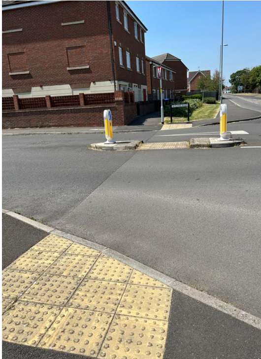
Photograph 6: Pedestrian infrastructure along Skylark Road junction
