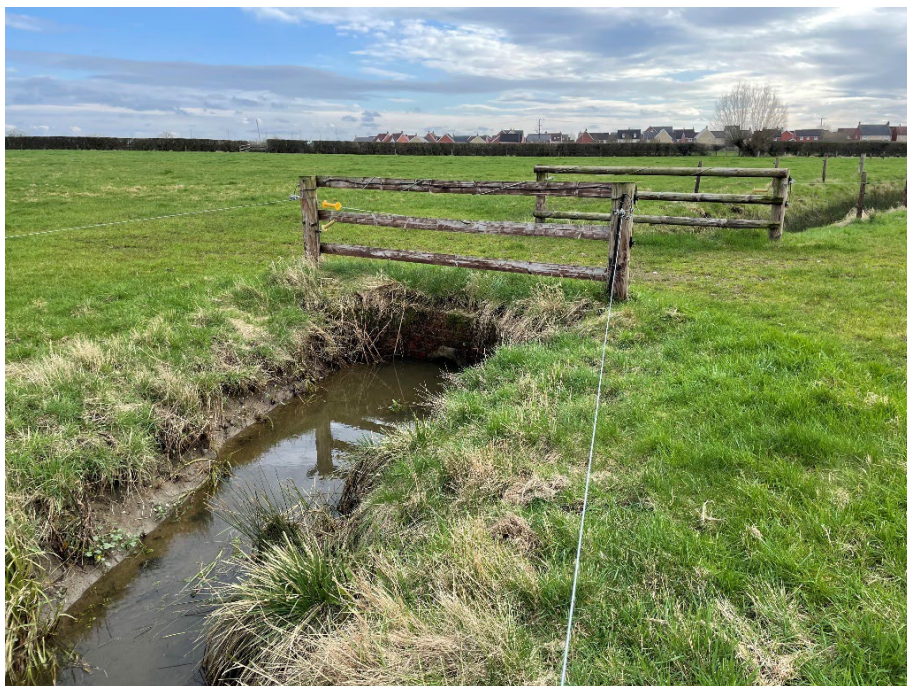
Photograph 4: South-facing view of one of the brick-built crossing points over the drainage channel.
