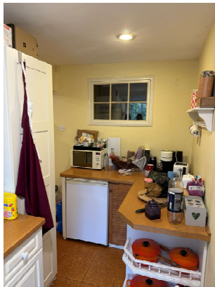
FIG 06 - Existing plasterboard wall as viewed from existing kitchen
