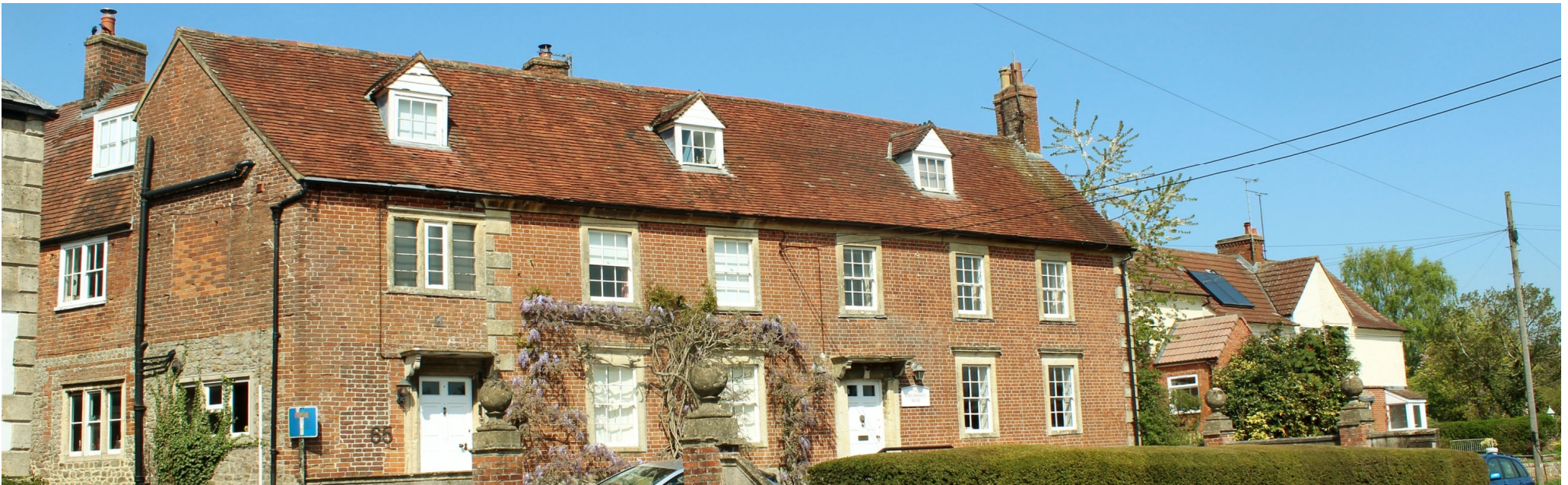
FIG 01 - Site Photo 01 (View of Wheelwrights House - Part of 65 & 63 High St., Chapmanslade)
