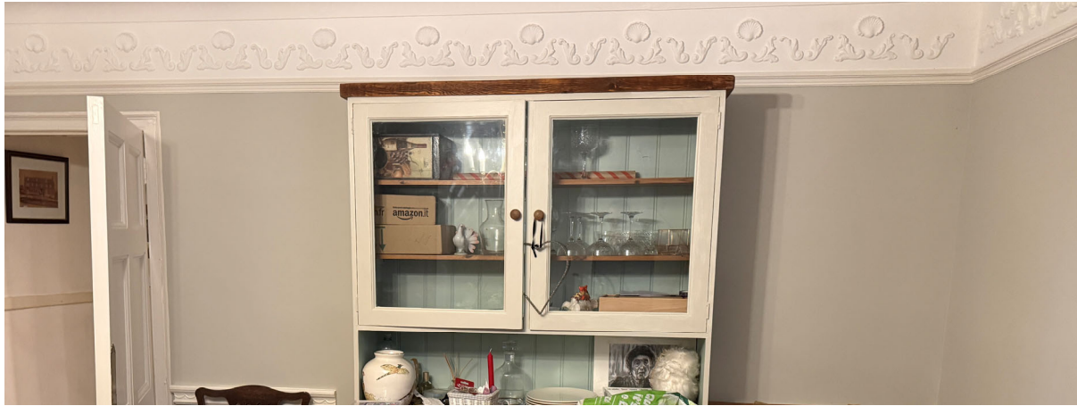
FIG 8 - Existing cornice as viewed from dining room. To be reinstated/ made good following works
