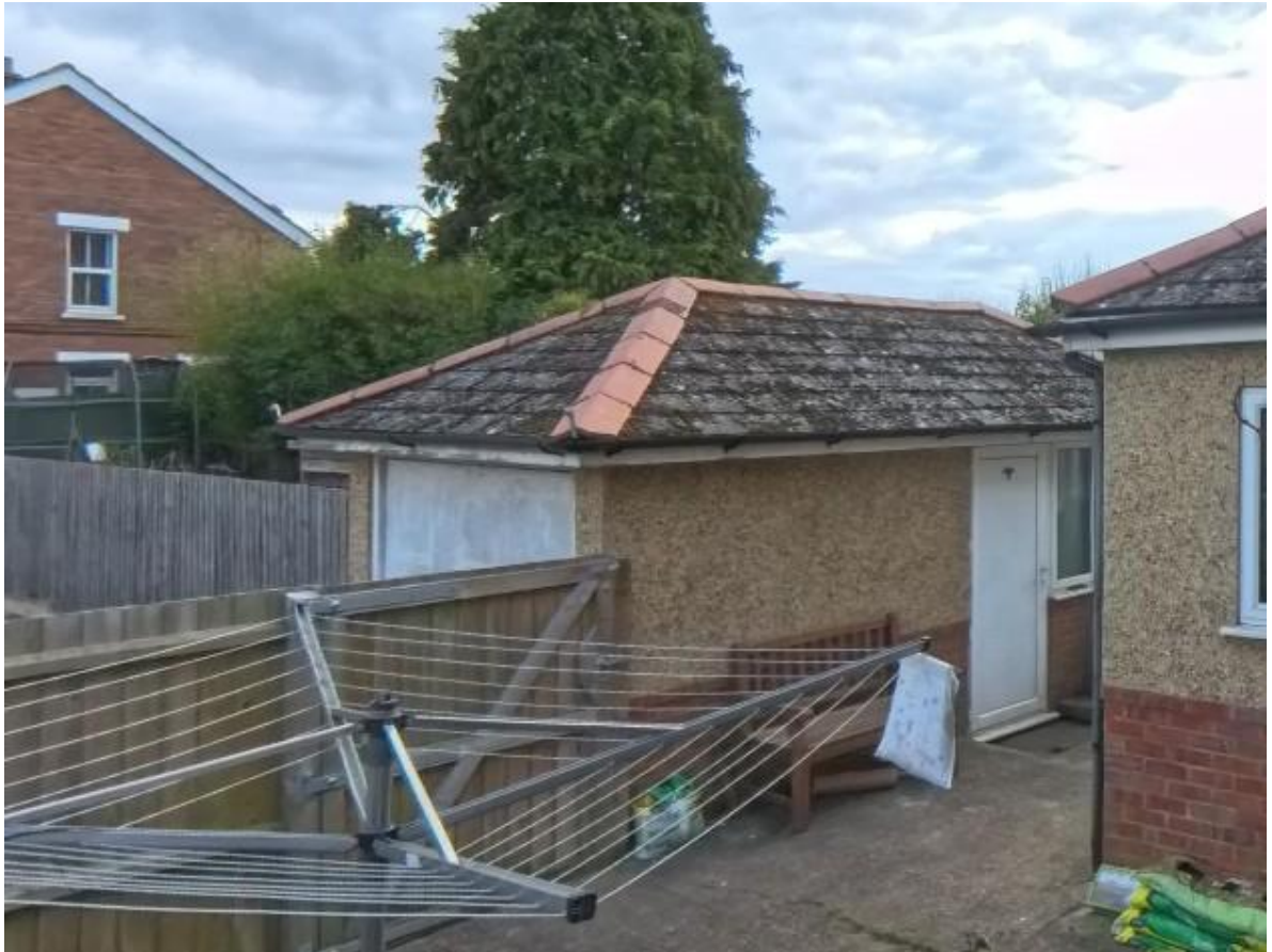
Figure 6. Garage looking southwest
