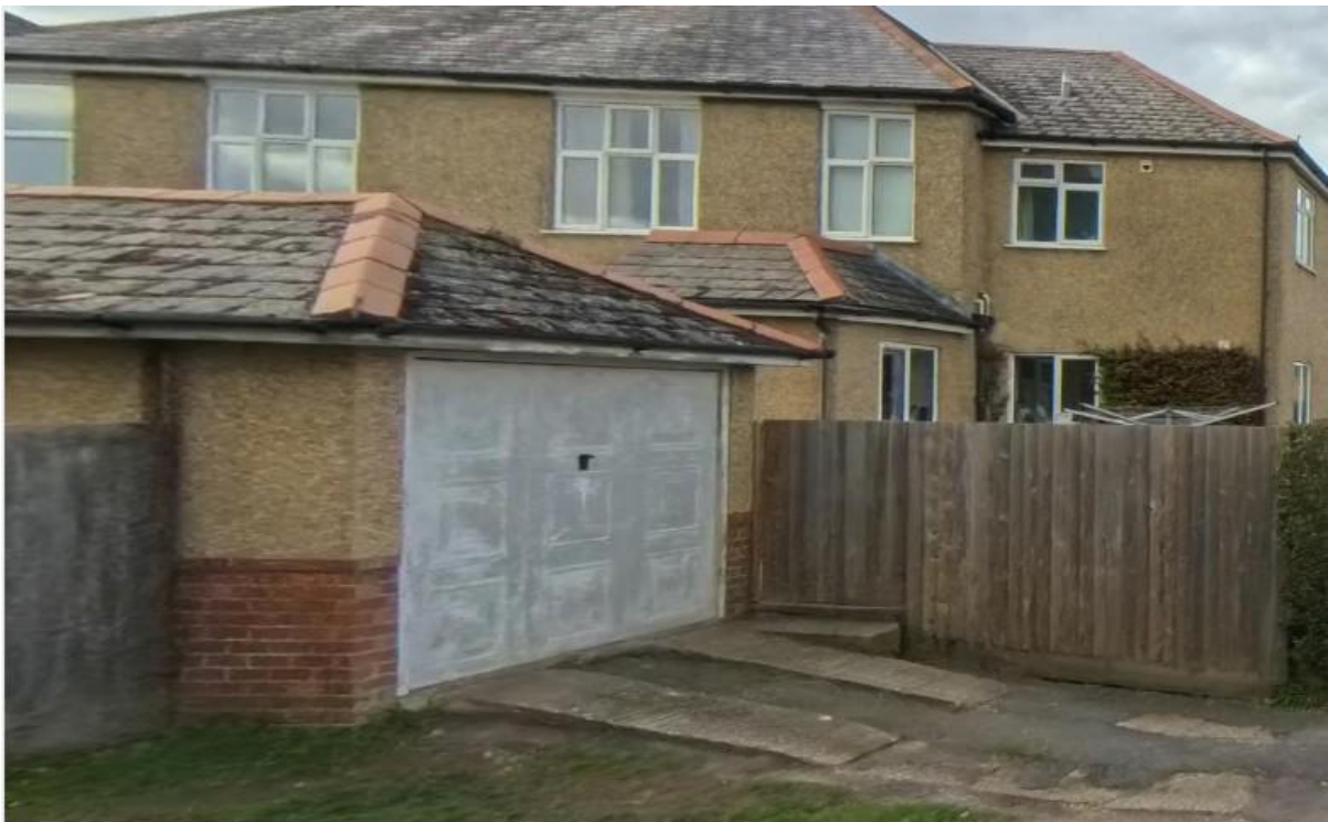
Figure 7. Garage looking northwest
