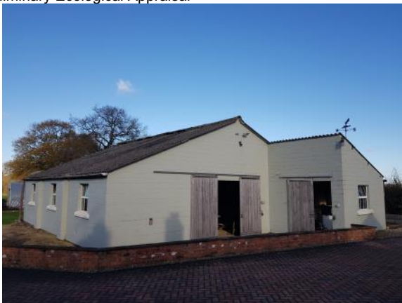
Photo 7: View of the surveyed building from the south.
