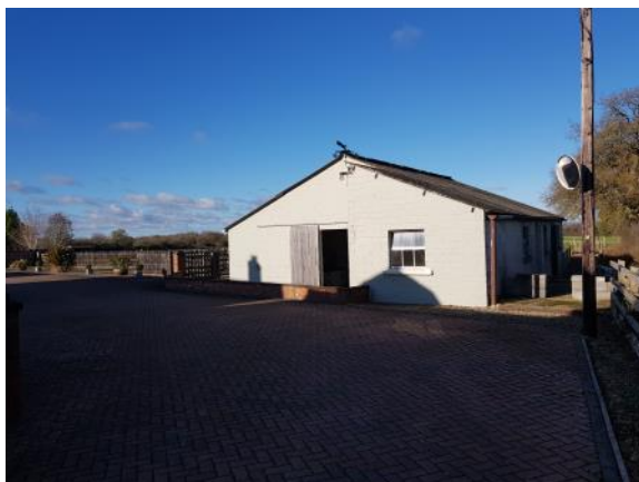
Photo 1: A view of the building and access driveway at the south of the site.
