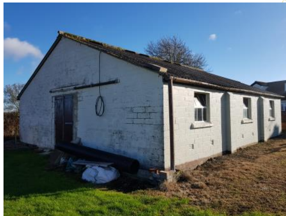
Photo 8: View of the surveyed building from the north-west.
