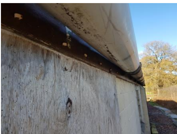
Photo 9: Well fitted gutter boards located at the eaves of the side elevations.
