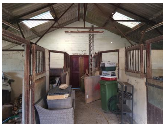
Photo 10: An internal view of the surveyed building.
