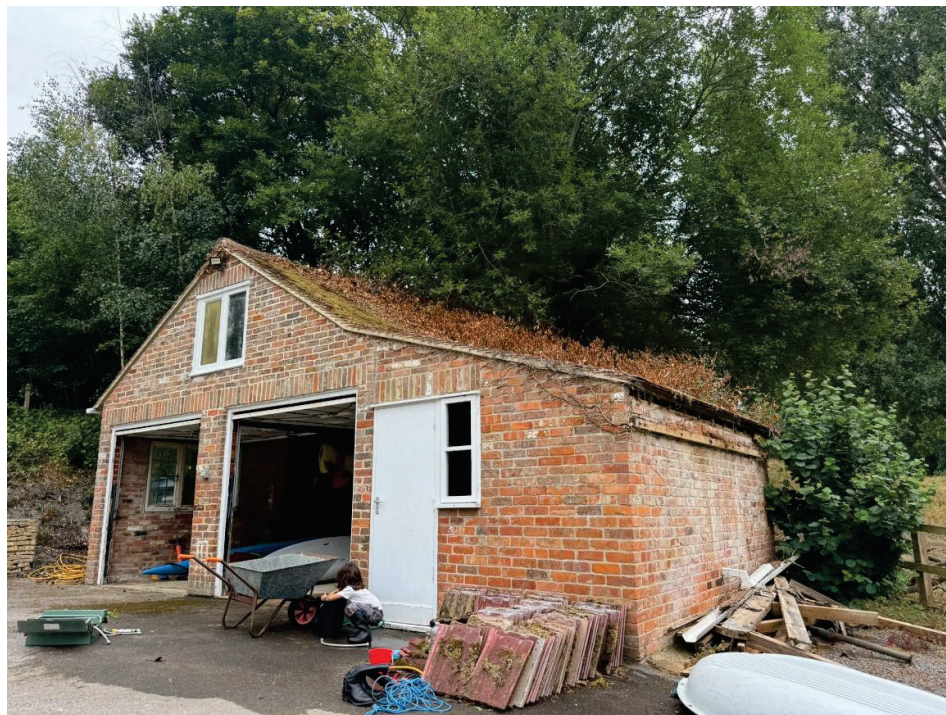
Plate 7: Northern and western elevation of the garage
