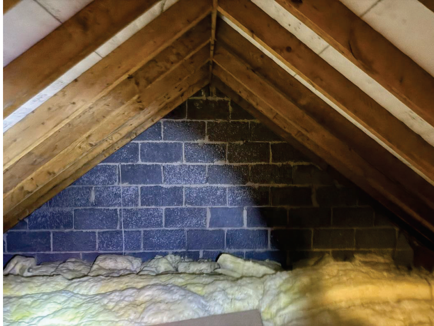
Plate A2: Roof void of Main Property
