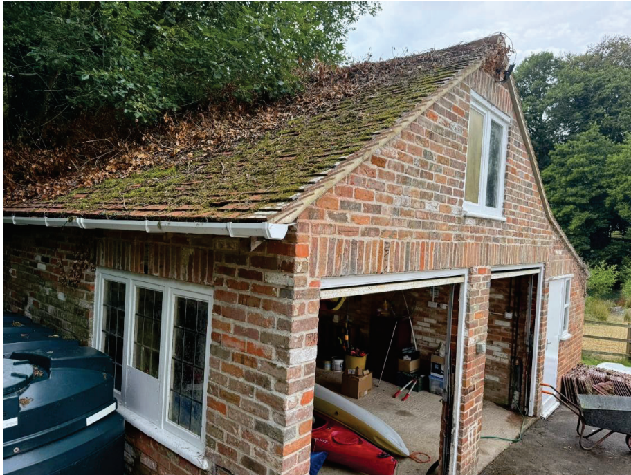
Plate A3: Northern and Eastern elevation of Garage
