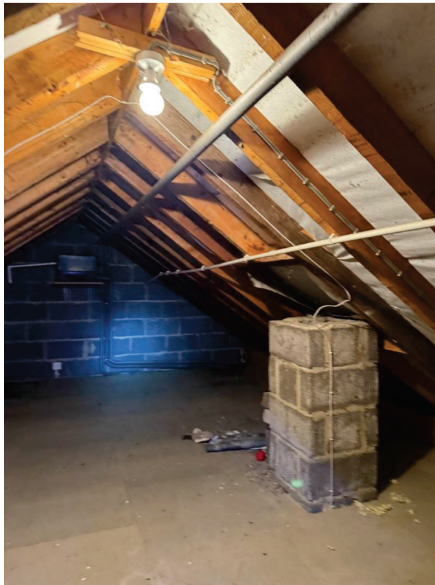
Plate A2: roof void of Main Property
