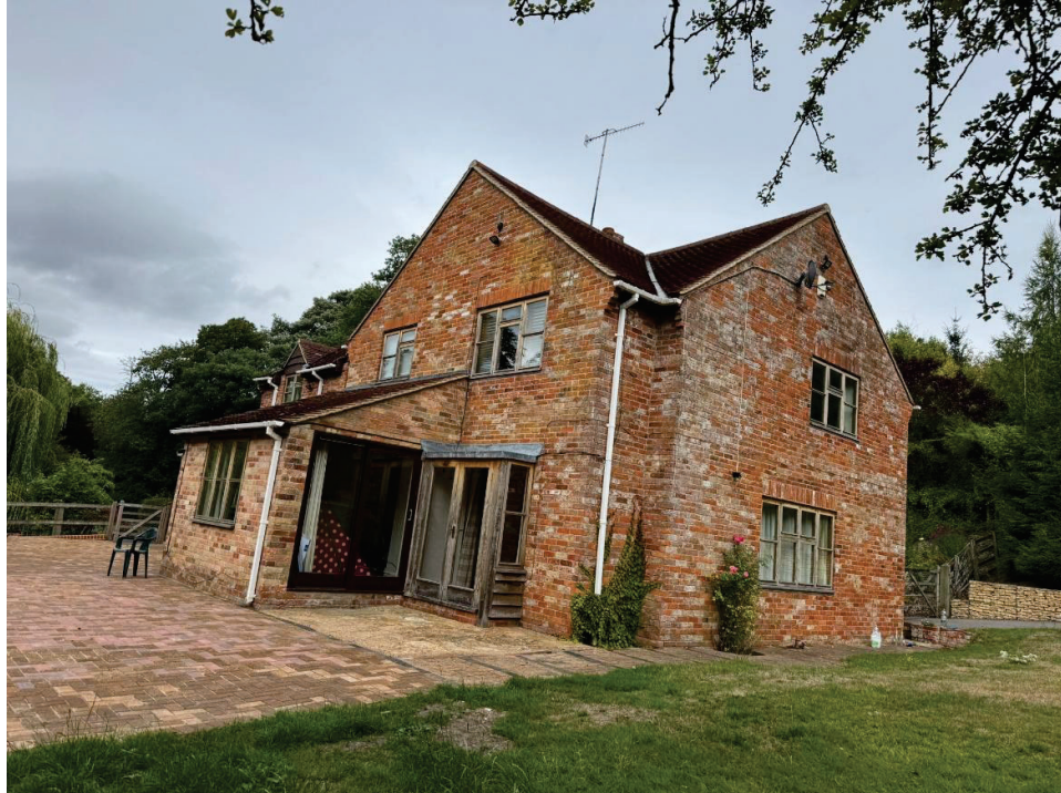
Plate 5: Southern and western elevation of property
