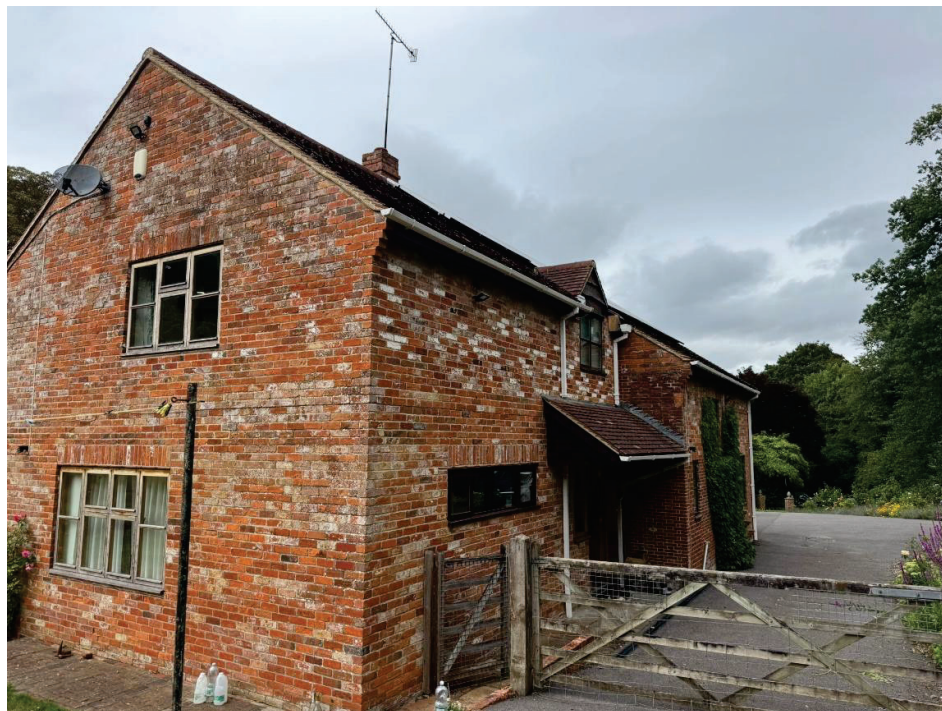
Plate 6: Southern and eastern elevation of property
