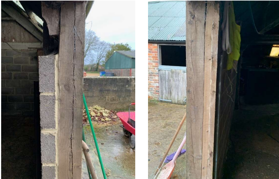
Fig 03 – indicating blockwork inner skin behind modern brickwork at north facing elevation. See fig 01 for location also.
