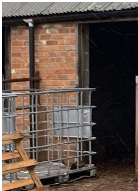
Fig 04 – indicating blockwork inner skin behind modern brickwork. At West facing elevation. See fig 02 for location also.
