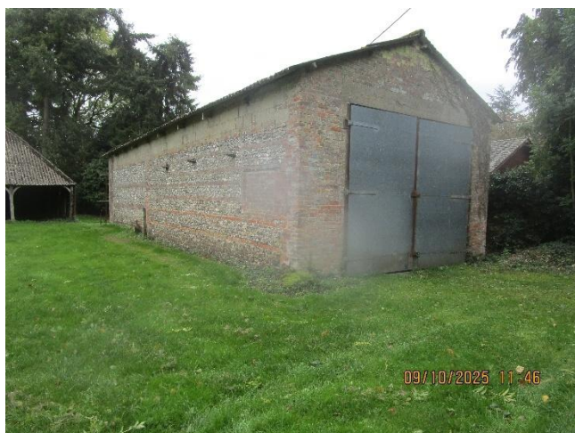
Photo 11 – Gaps between in the brickwork and gaps between the roof and wall at the gable end, and, Photo 12 - Open eaves, with gaps between the wall top and roof overhang
