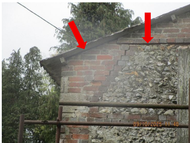
Photo 11 – Gaps between in the brickwork and gaps between the roof and wall at the gable end, and, Photo 12 - Open eaves, with gaps between the wall top and roof overhang
