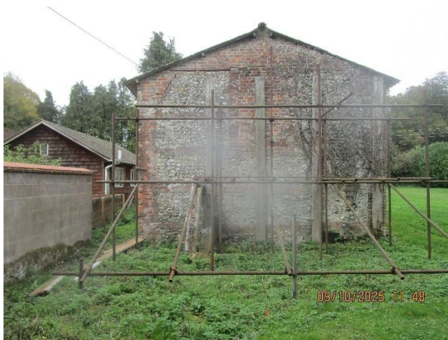
Photo 11 – Gaps between in the brickwork and gaps between the roof and wall at the gable end, and, Photo 12 - Open eaves, with gaps between the wall top and roof overhang
