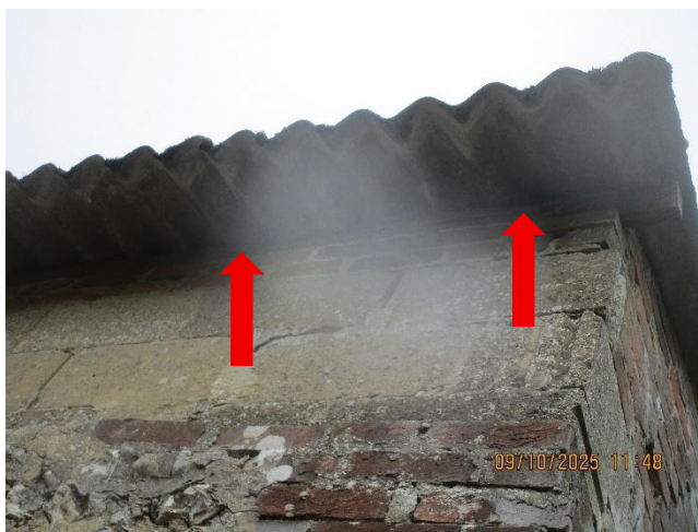
Photo 11 – Gaps between in the brickwork and gaps between the roof and wall at the gable end, and, Photo 12 - Open eaves, with gaps between the wall top and roof overhang
