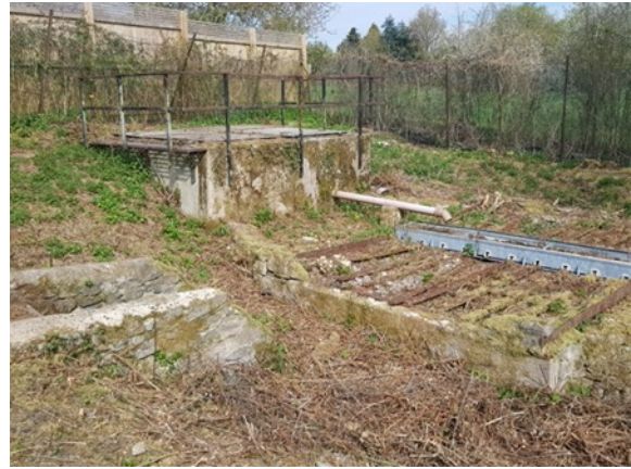
Photo 8: Concrete remnants of former sewage works.
