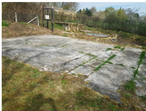
Photo 6: u1b concrete hardstanding.
