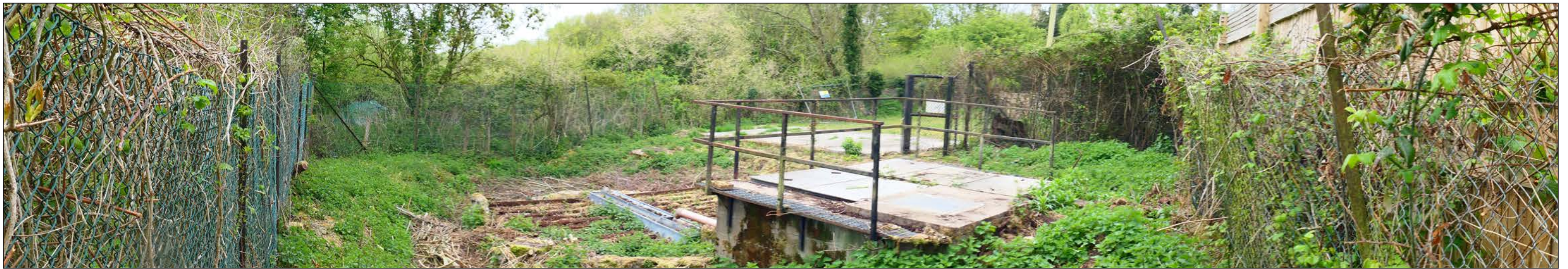
View h. Looking south east across the Site 25-04-25
