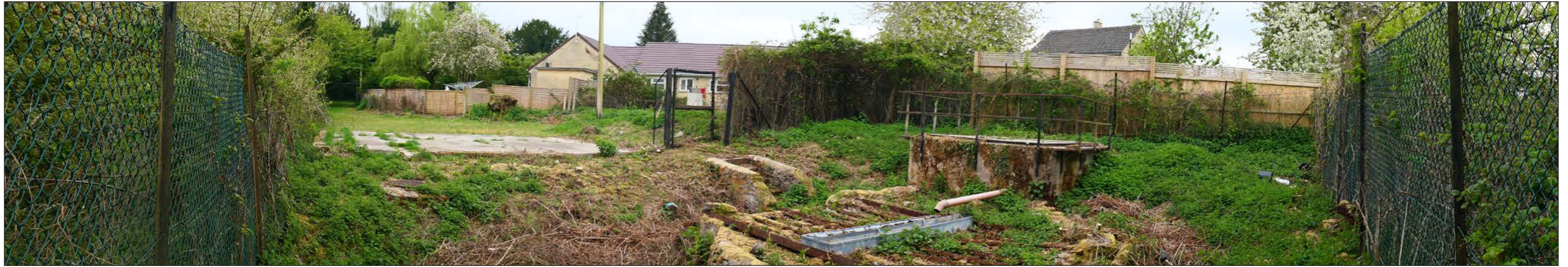
View g. Looking south west across the Site 25-04-25
