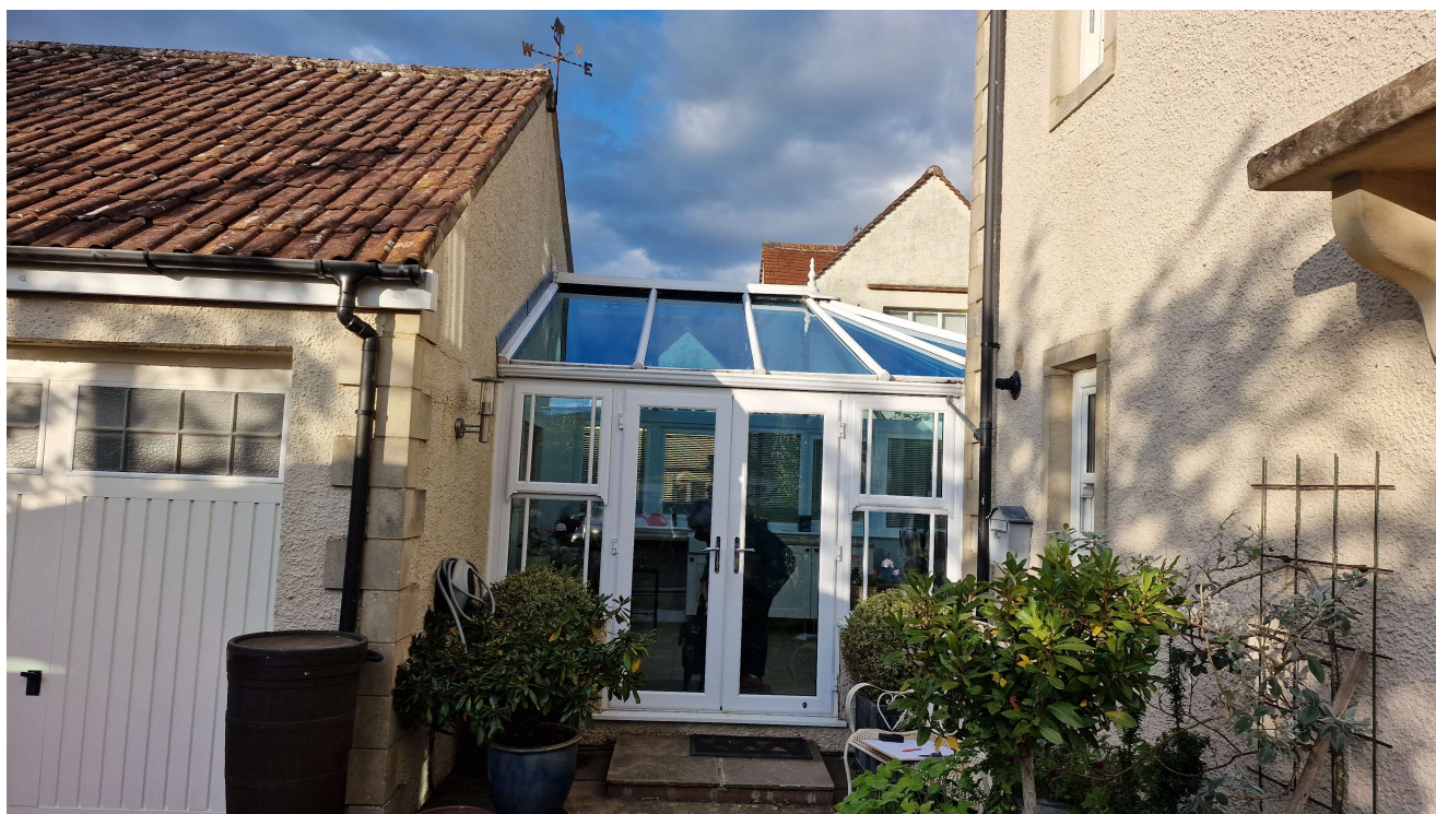
View of conservatory linking to existing front garage from south, main house to right.
