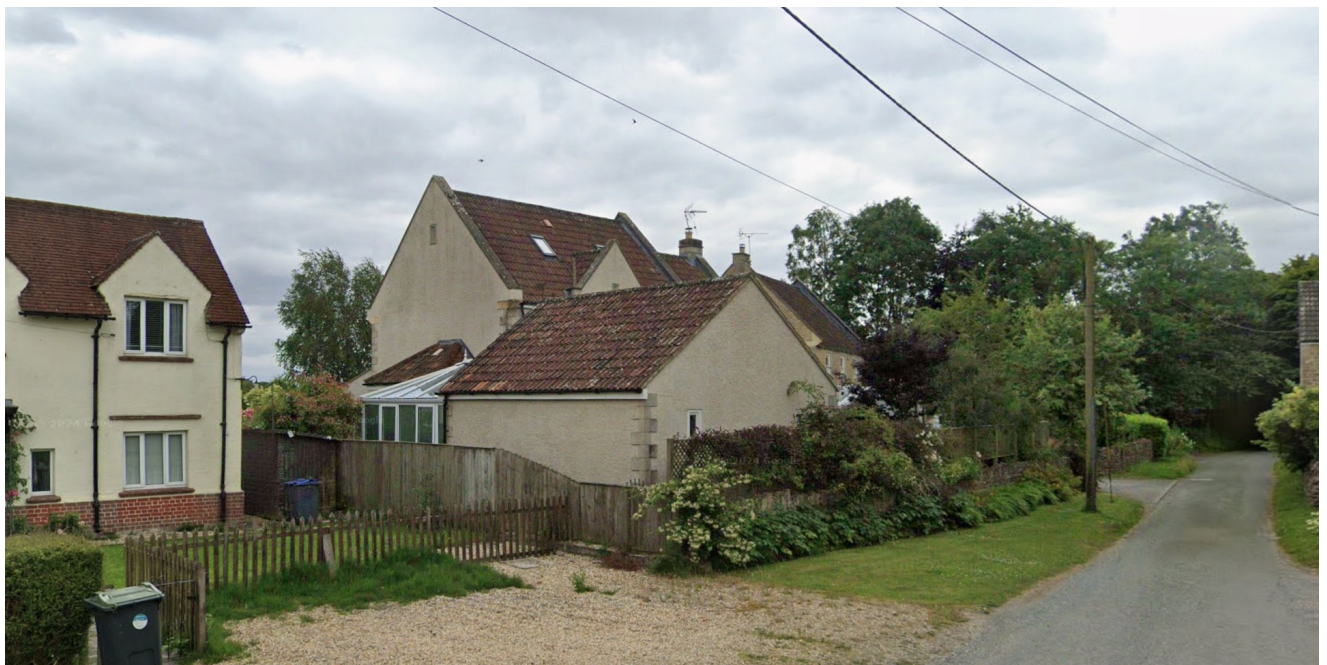
Holly House from north of site approach, in front garage with conservatory to rear connects to side of house
