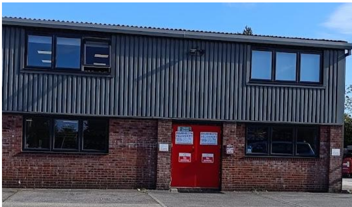
Extract 8: Existing buildings in Industry Park (brick with grey cladding above)
