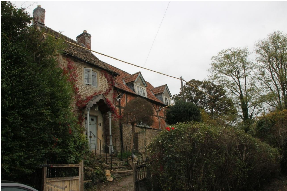
Photograph 1: showing a view of the target building (front elevation of the house)
