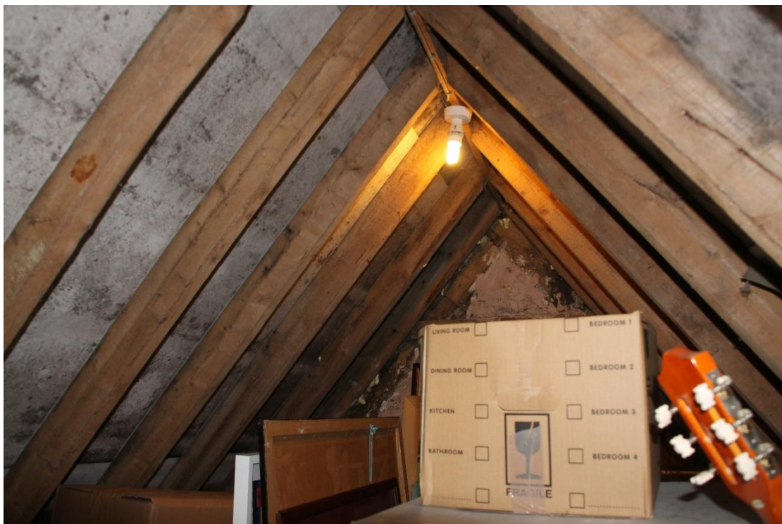
Photograph 3: showing a view of loft space above the original cottage to the north of the building
