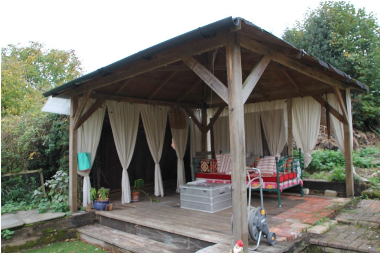
Photograph 7: showing a view of the wooden pergola
