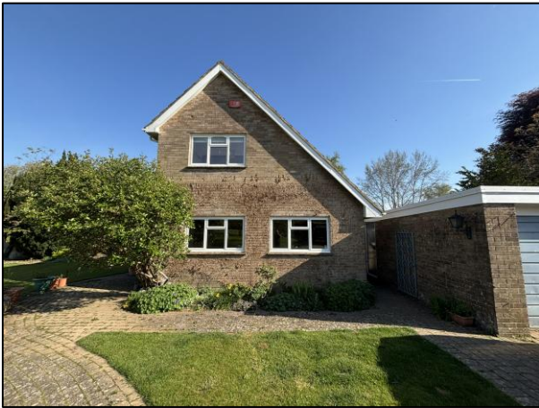
South elevation with no entrance visible
