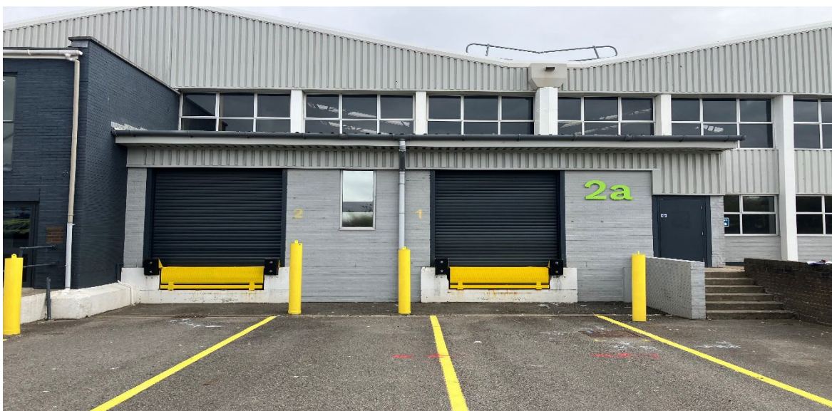
Fig. 3: Existing front elevation of dock level loading bay doors of Unit 2A
