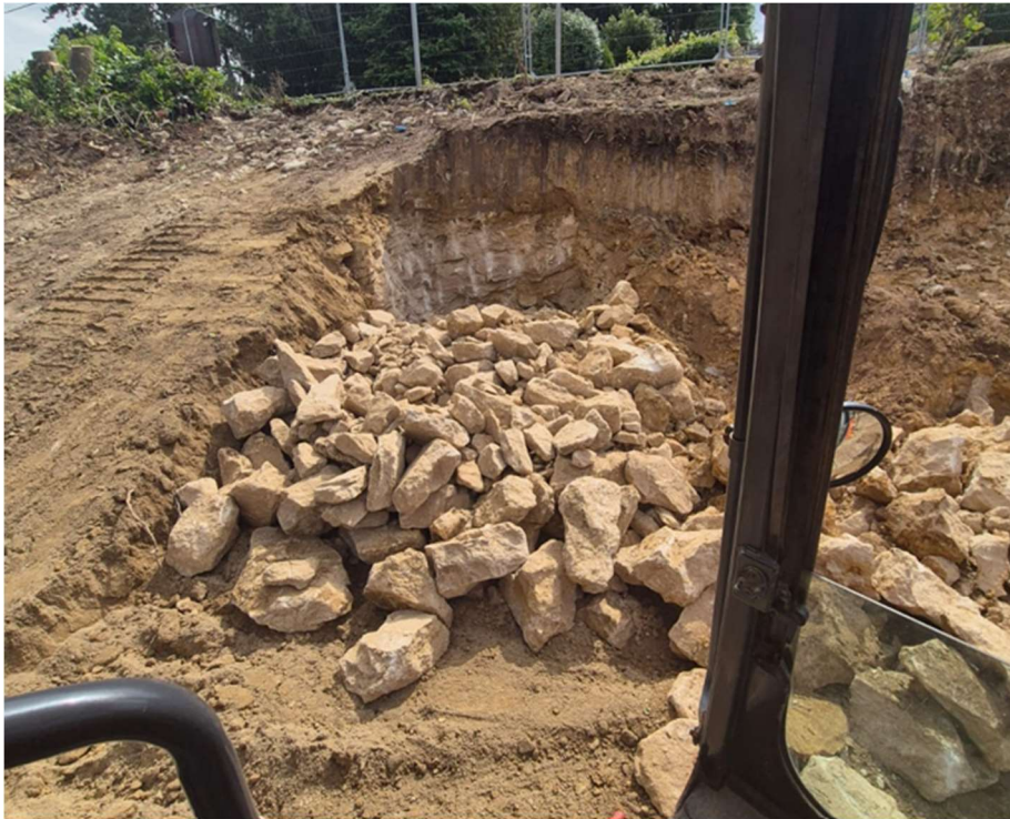
Plate 2.2: Excavated limestone boulders, as part of plot preparation, awaiting crushing.
