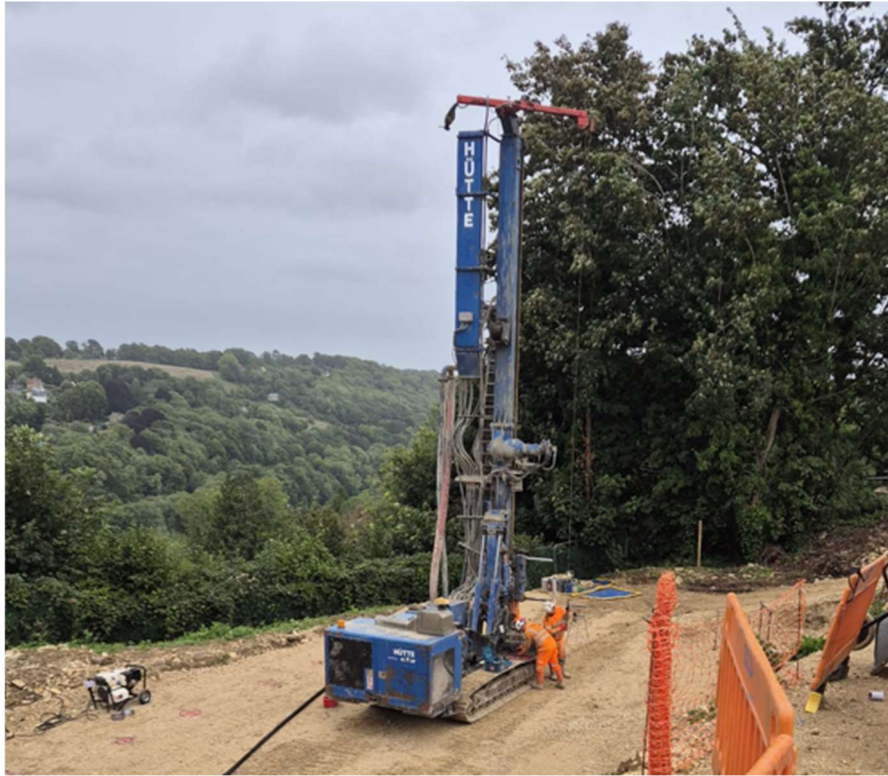
Plate 2.5: Installation of Odex piles by GeMech.
