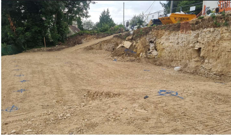
Plate 2.1: Image facing South, with position of piles marked on ground. Intact weathered limestone forming the face of the excavation
