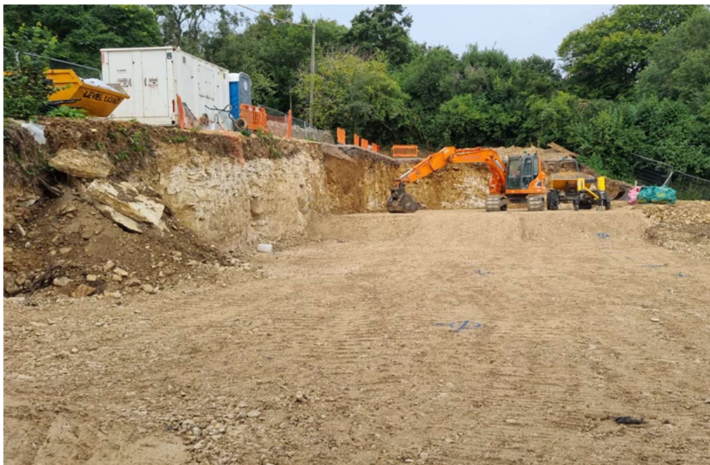
Plate 2.4: Exposed face of cutting, indicating localised historical surface excavation of limestone. No evidence of below ground workings.
