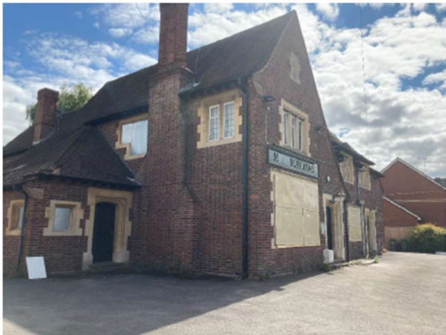
Photograph 1- North and west face of pub
