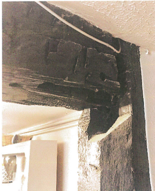
Figure 10 Detail of the junction between the cross-beam ceiling and a former door post against the southern wall of the kitchen showing the Mason's mitre to the post and a void mortise and stave hole in the soffit of the beam.
