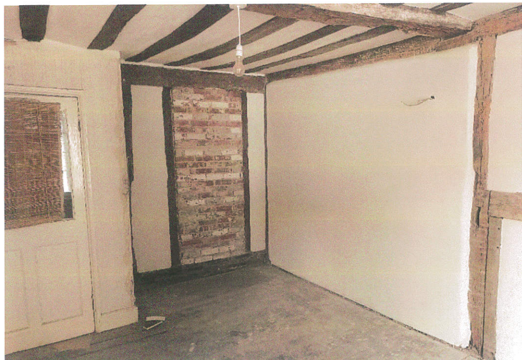
Figure 14 The western rear room at first floor level, facing south-west.
