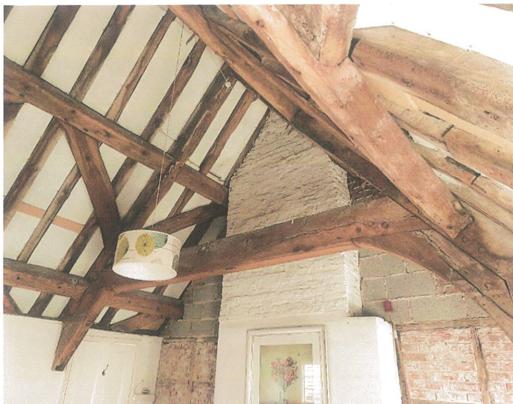
Figure 16 The roof truss exposed within the second-floor front room.
