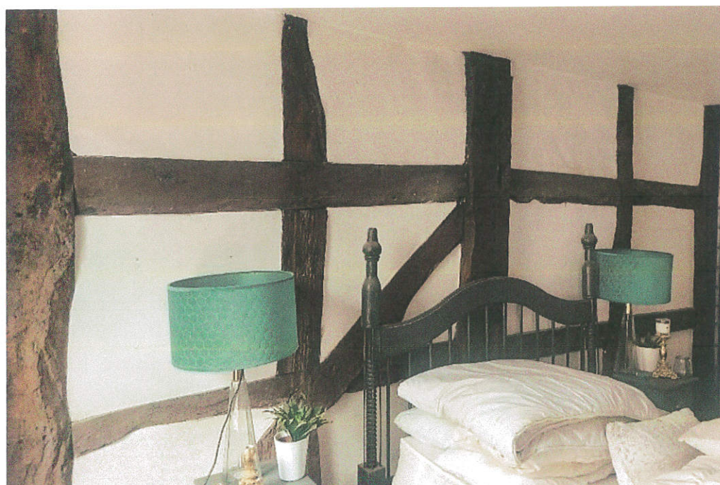
Figure 12 The framing of the west wall of the front bedroom at first floor level.
