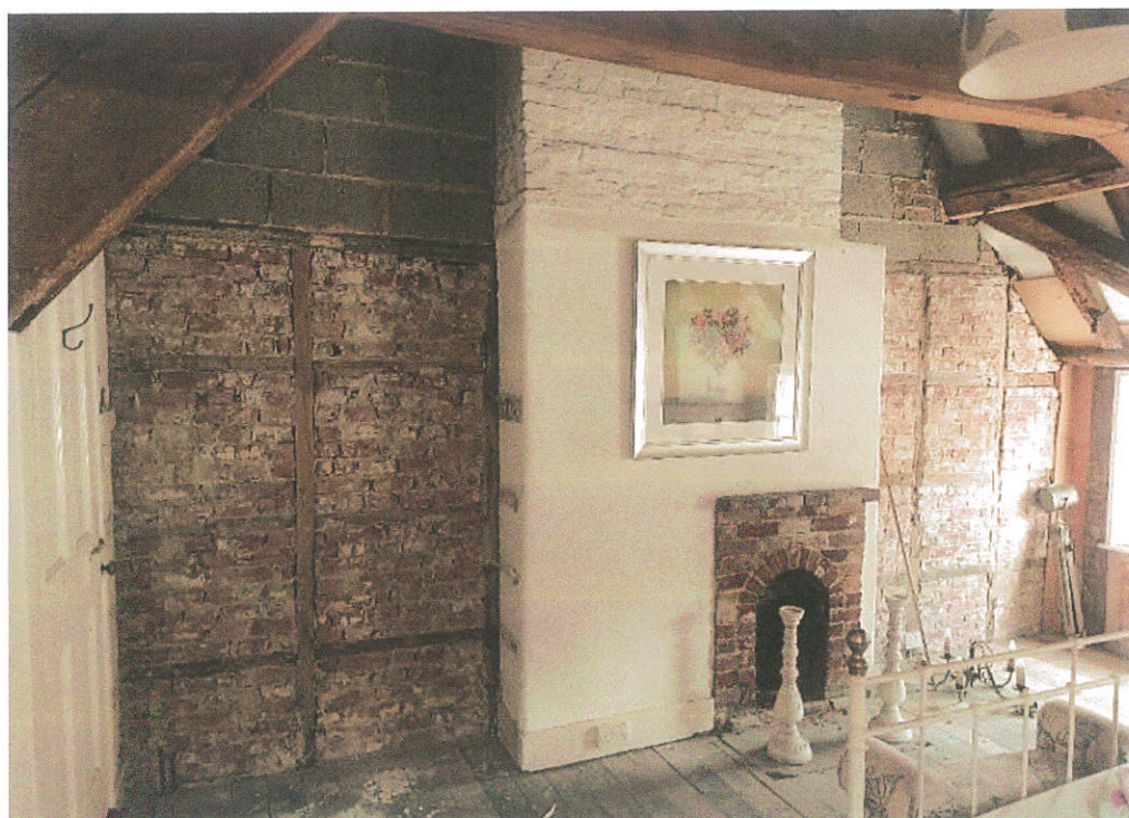
Figure 17 The east wall of the front second floor room.
