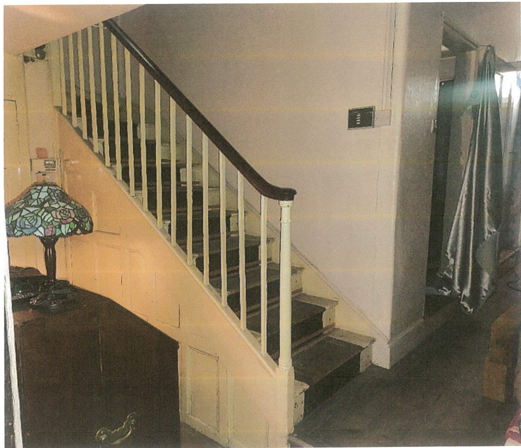
Figure 7 The staircase to the first floor.
