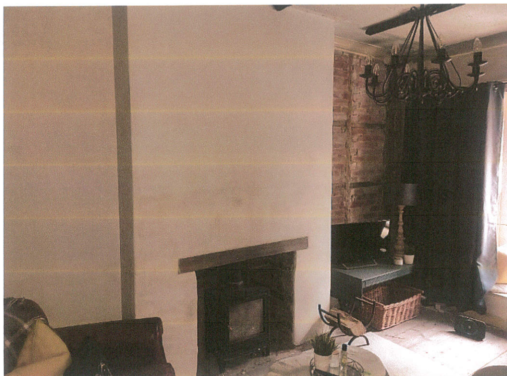
Figure 6 The chimney breast and timber-laced partition wall between the two houses within the front principal room.
