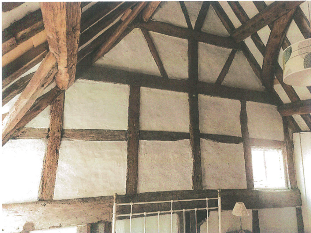
Figure 15 The wall framing of the west wall of the second-floor room.
