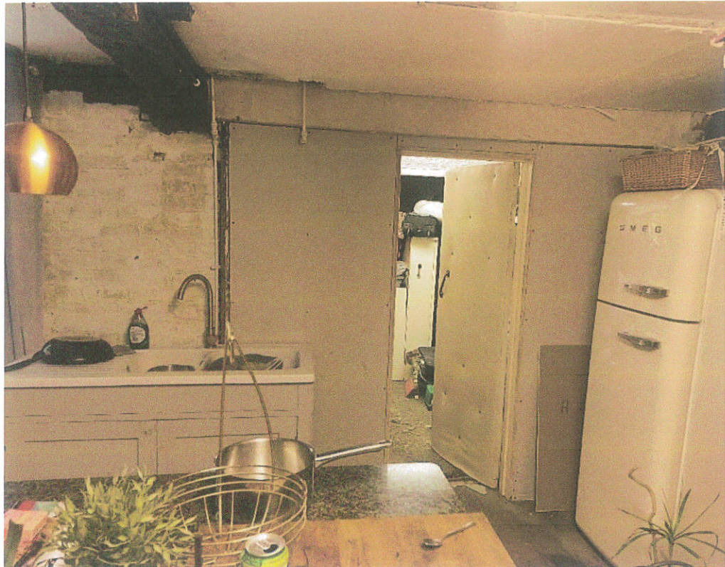
Figure 9 The eastern part of the north wall where a large opening has been infilled with modern stud and plasterboard.
