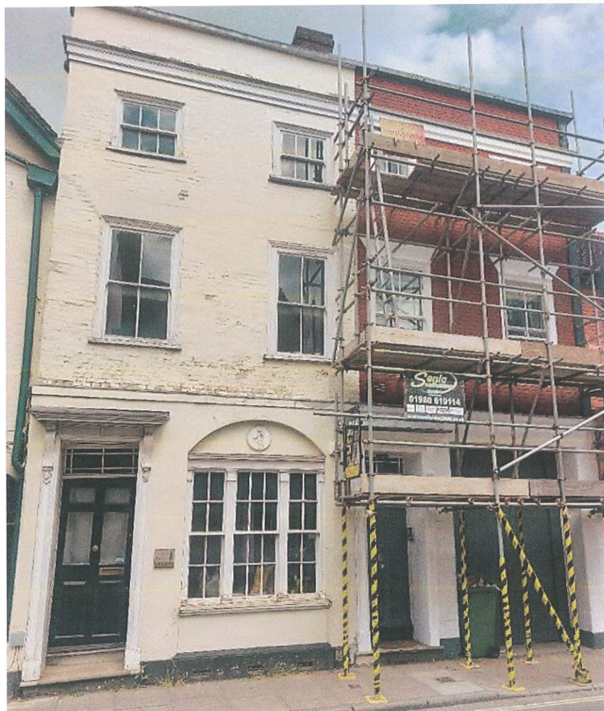
Figure 2 The front elevation is of No. 82 and No. 84 (the building to the left).
