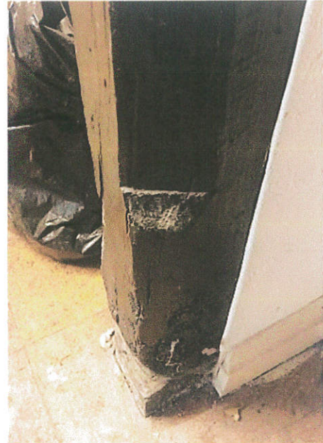
Figure 11 Detail of the stopped chamfer to the former door post set against the south wall of the kitchen.
