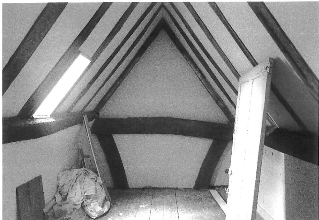
Figure 18 The collar to the truss at the west end of the western room at attic level.
