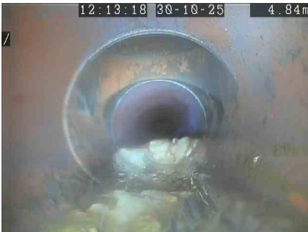
1d9ef36b-8513-4ef1-9a2e-1d5fa7eaac4c.png, 00:01:19, 4.84 m Junction at 12 o'clock, 100mm dia
