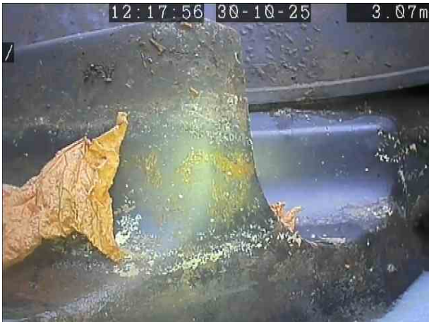
97d349a2-27e7-418f-8d53-4b90eef1f823.png, 00:00:25, 3.07 m Finish node, manhole, reference: I/C2
