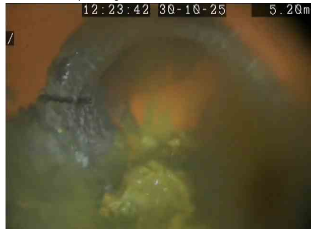
5101a980-e25d-470d-91eb-95607be5ca5e.png, 00:00:23, 5.20 m Finish node, manhole, reference: U/S, INT SVP
