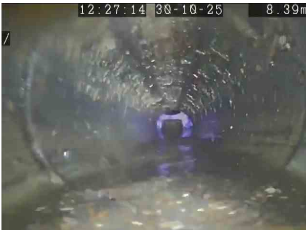
b17f079f-17da-4e3a-bfd1-0122a7252581.png, 00:00:27, 8.39 m Water level, 20% of the vertical dimension
