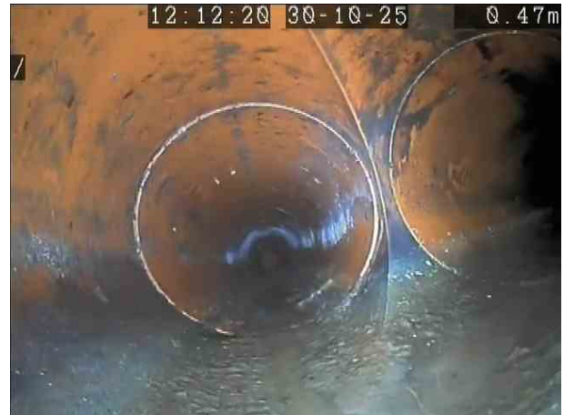
4c76dd7a-af2e-46fe-b2d4-420cf6fa053a.png, 00:00:21, 0.47 m Junction at 2 o'clock, 100mm dia
