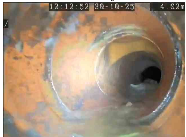
c90c9753-df6d-44ef-897b-b0f78d7fdea2.png, 00:00:53, 4.02 m Line deviates right
