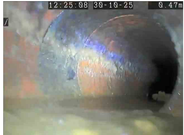
9aaeda33-3aef-4afb-8320-1165545c9bd4.png, 00:00:12, 0.47 m Line deviates right
