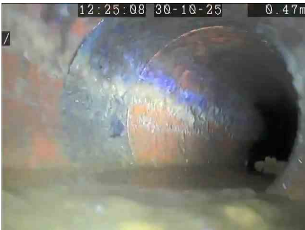
5a3a6218-ea7d-47a9-8565-31facc8db93a.png, 00:00:12, 0.47 m Water level, 10% of the vertical dimension
