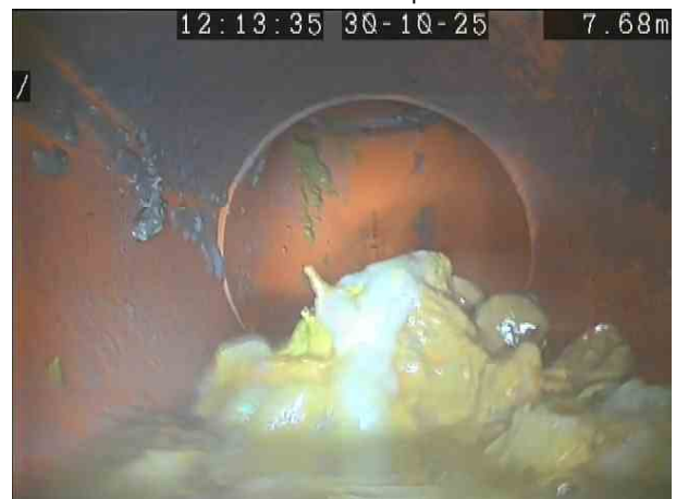
8e68ea9b-c662-4732-810d-25dc741879a5.png, 00:01:36, 7.68 m Finish node, manhole, reference: IWP
