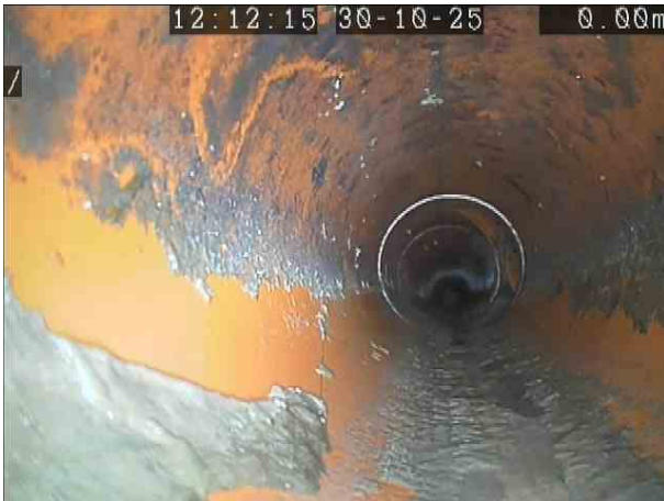
800db7ab-f025-4438-81c6-8e217f609b8e.png, 00:00:16, 0.00 m Start node, manhole, reference: VC1
