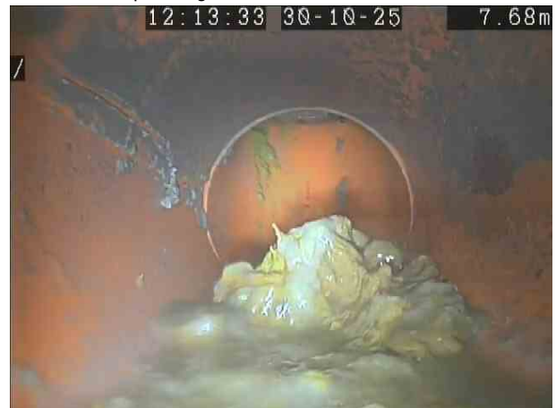
89bca9b3-2d64-4ca4-8399-16b183d1cbf3.png, 00:01:34, 7.68 m Line deviates up
