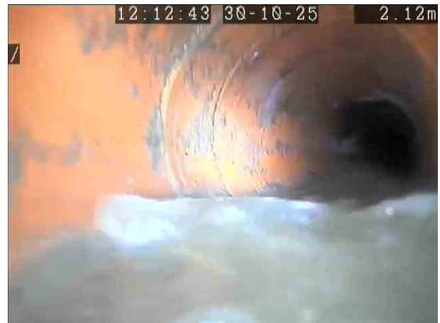
05b06225-1e5a-4a49-b3e5-6bbf545e327d.png, 00:00:44, 2.12 m Line deviates right
