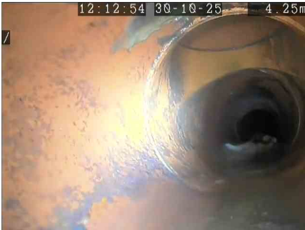
77afa18b-d1a3-4451-a0ec-ca148182b4ef.png, 00:00:54, 4.25 m Junction at 12 o'clock, 100mm dia
