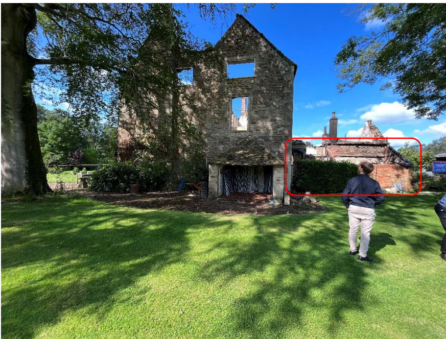
Fig. 01. East Elevation capturing modern lean-to extensions built from brickwork (marked in red).
