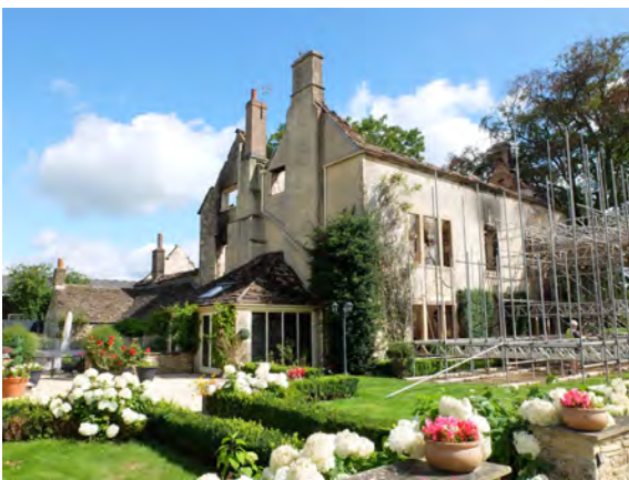
Fig.18 Farmhouse viewed from west
