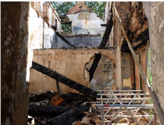
Fig.28 &29 View through the main range from west
