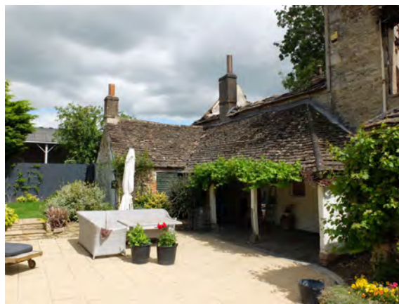
Fig.19 West courtyard intact
