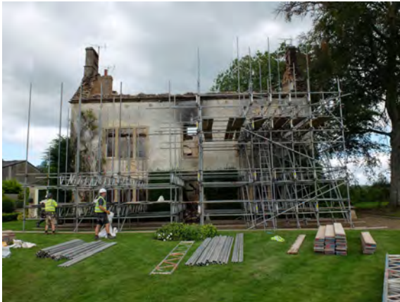
Fig.20 Front elevation as scaffolding erected to prop front.
