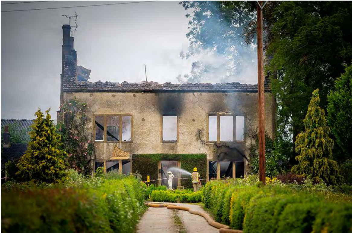
Fig.17 June 1 st 2023 Source: https://www.wiltshire999s.co.uk/grade-listed-farmhouse-destroyed-blaze/
