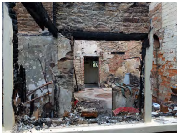
Fig.25 Adjoining rear range
