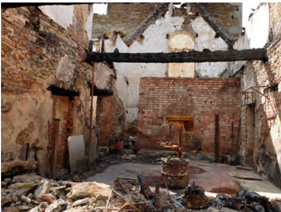
Fig.24 View into rear range from north
