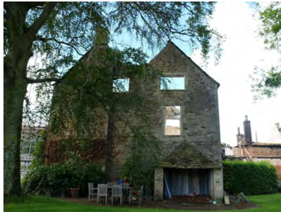
Fig.21 East elevation with lean-to shelter and hipped roof
