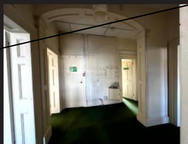
FIG.9 Central Lobby area
