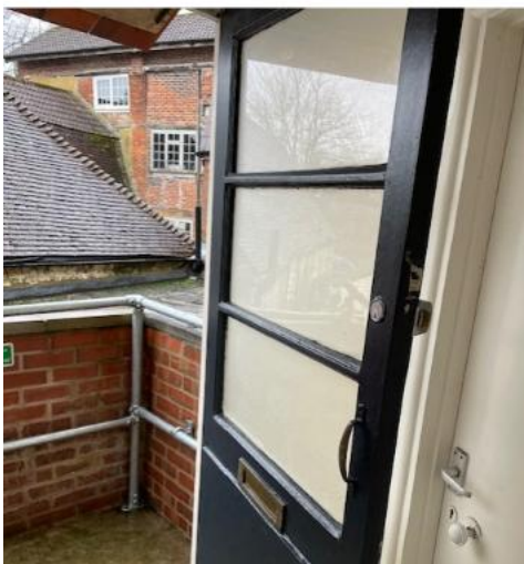
Rear first floor door – access to flats
