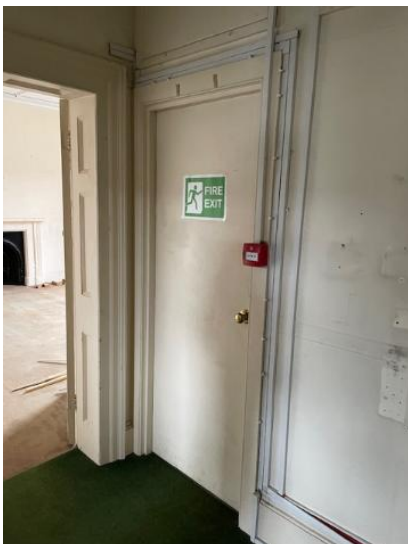
Door to stairwell
