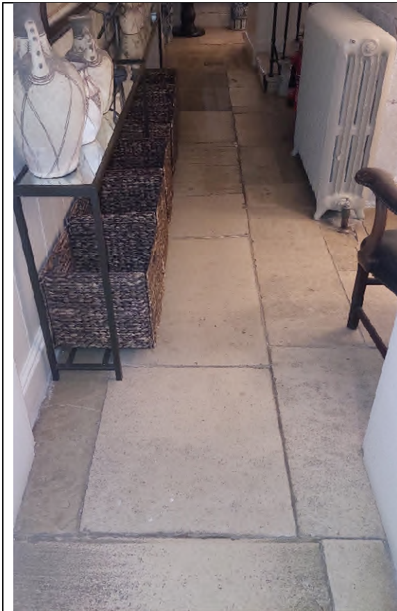
Photo 21 Corridor to NW Stairs, B46
