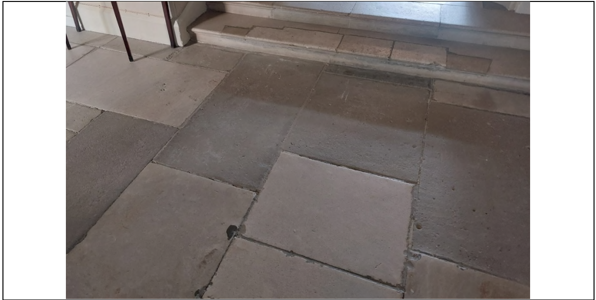
Photo 20 Lower East Cloister
