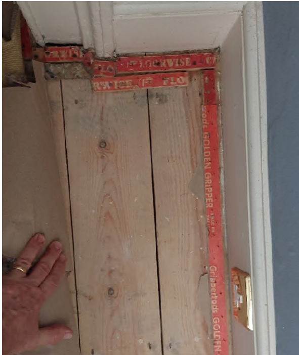
Photo 13 Lower S Cloister 4 showing softwood floorboards beneath carpet
