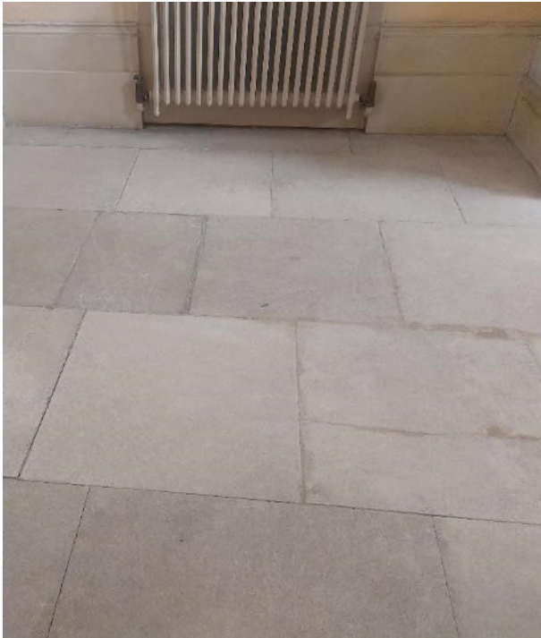
Photo 39 Entrance Hall, G15
