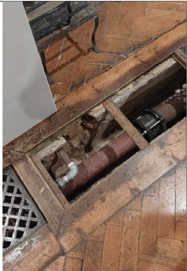
Photo 22 Laundry, B33. Pipe in trench with metal grille over and parquet floor
