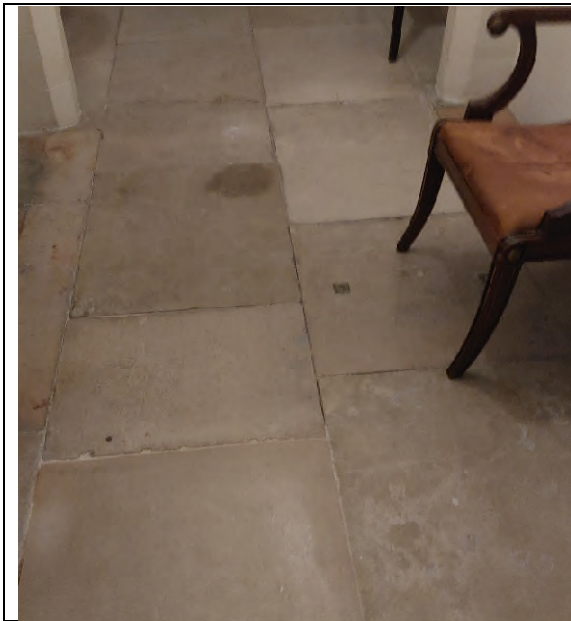
Photo 16 S of Gothic stair, B1
