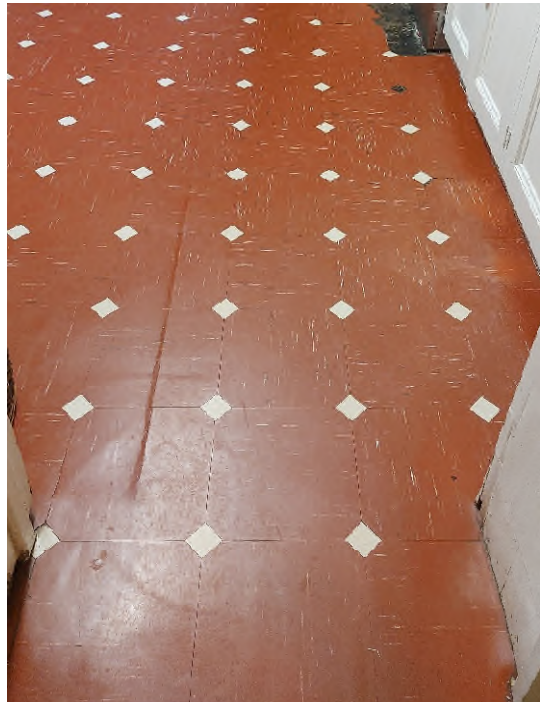
Photo B4 Service Kitchen B26
